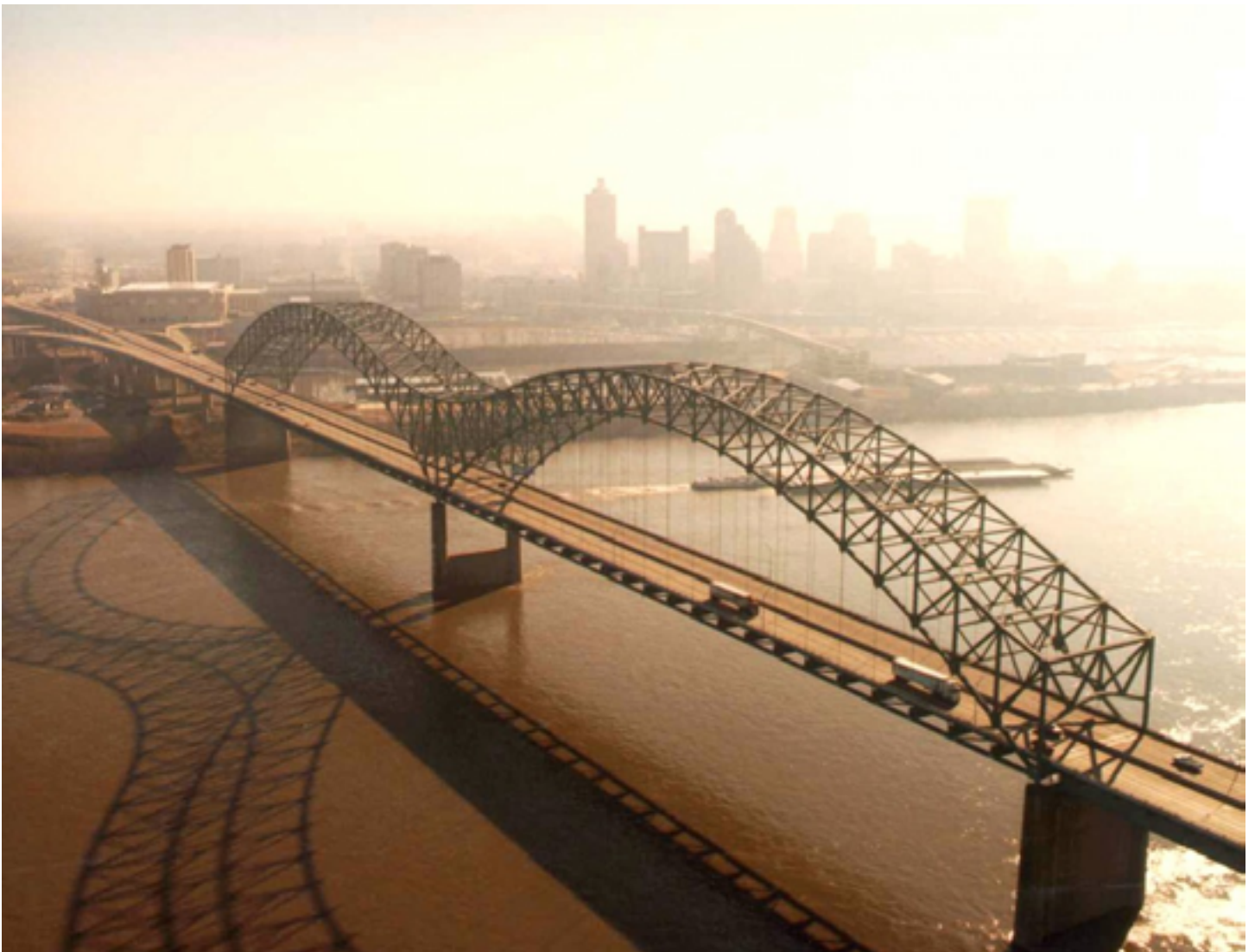
Aerial view of the Hernando de Soto Bridge across the Mississippi River between Memphis, Tennessee and West Memphis, Arkansas, USA. The bridge was opened in 1973 and carries six lanes of Interstate 40 across the river. View is from the Arkansas side to the east-southeast across the river to Memphis. Photographer Larry Donald, U.S. Army Corps of Engineers.
