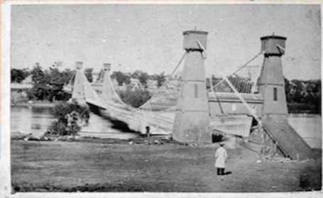
First Suspension Bridge 3
