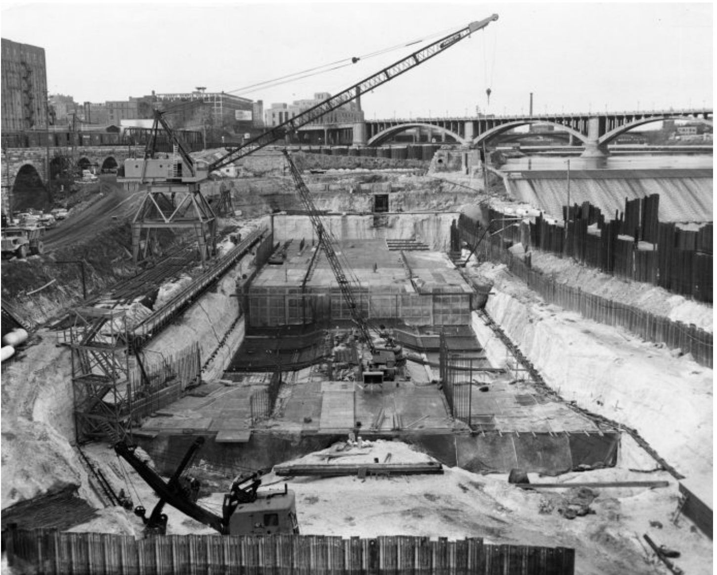
Figure 3. Construction of the Upper St. Anthony Falls lock, 1960. The current horseshoe-shaped hydro-electric dam, completed in 1963, is 49 feet in height (US Army Corps of Engineers 2016a). Photo by Dale L. Sperline, US Army; courtesy of the Minnesota Historical Society.
