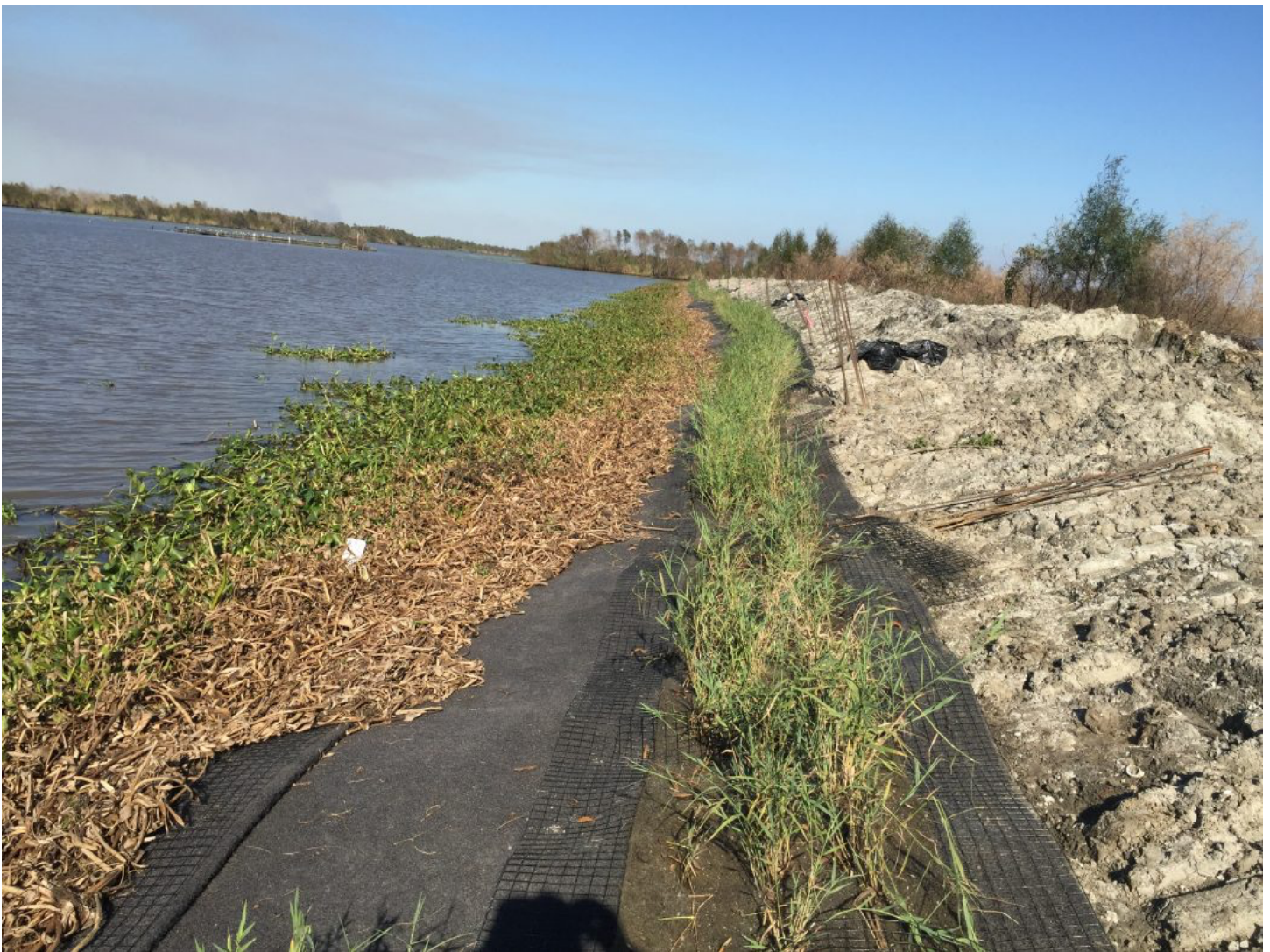
EcoShield in the midst of installation. Courtesy America's WETLAND Foundation.
