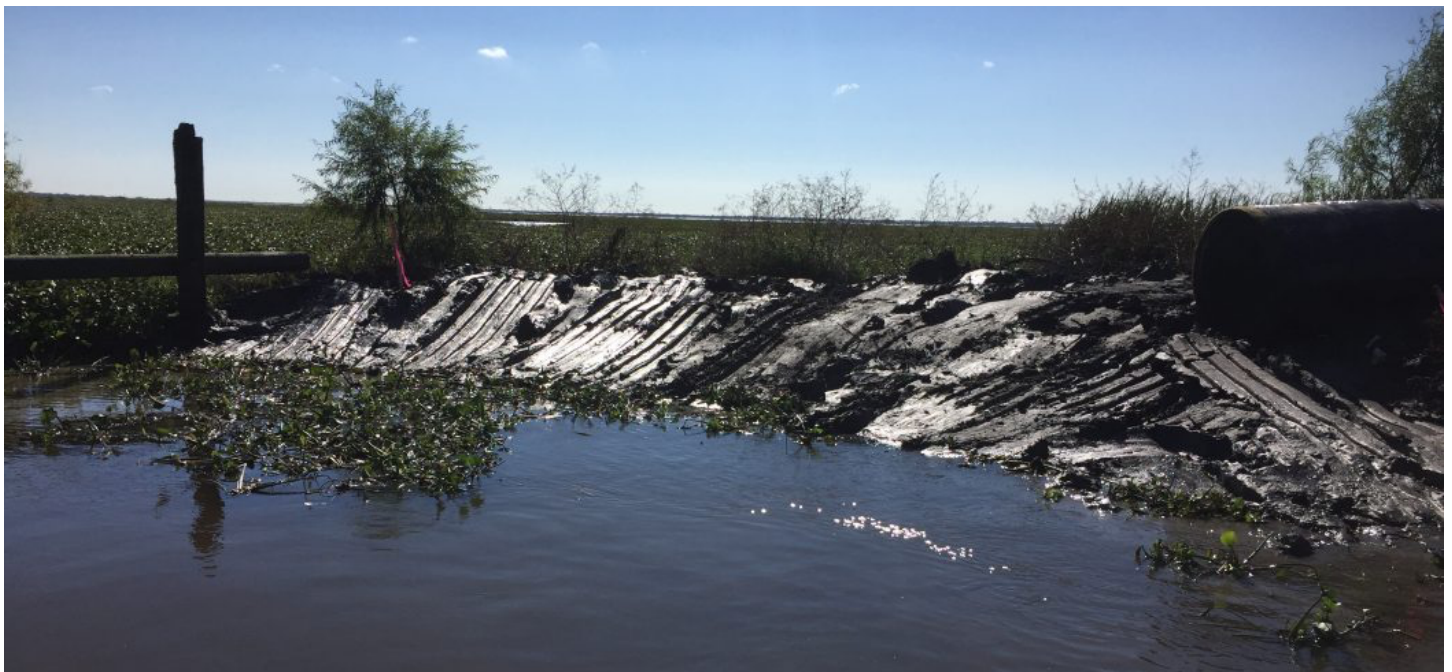
Newly created berm, ready for the installation of Vegetated EcoShield™. Courtesy America's WETLAND Foundation.
