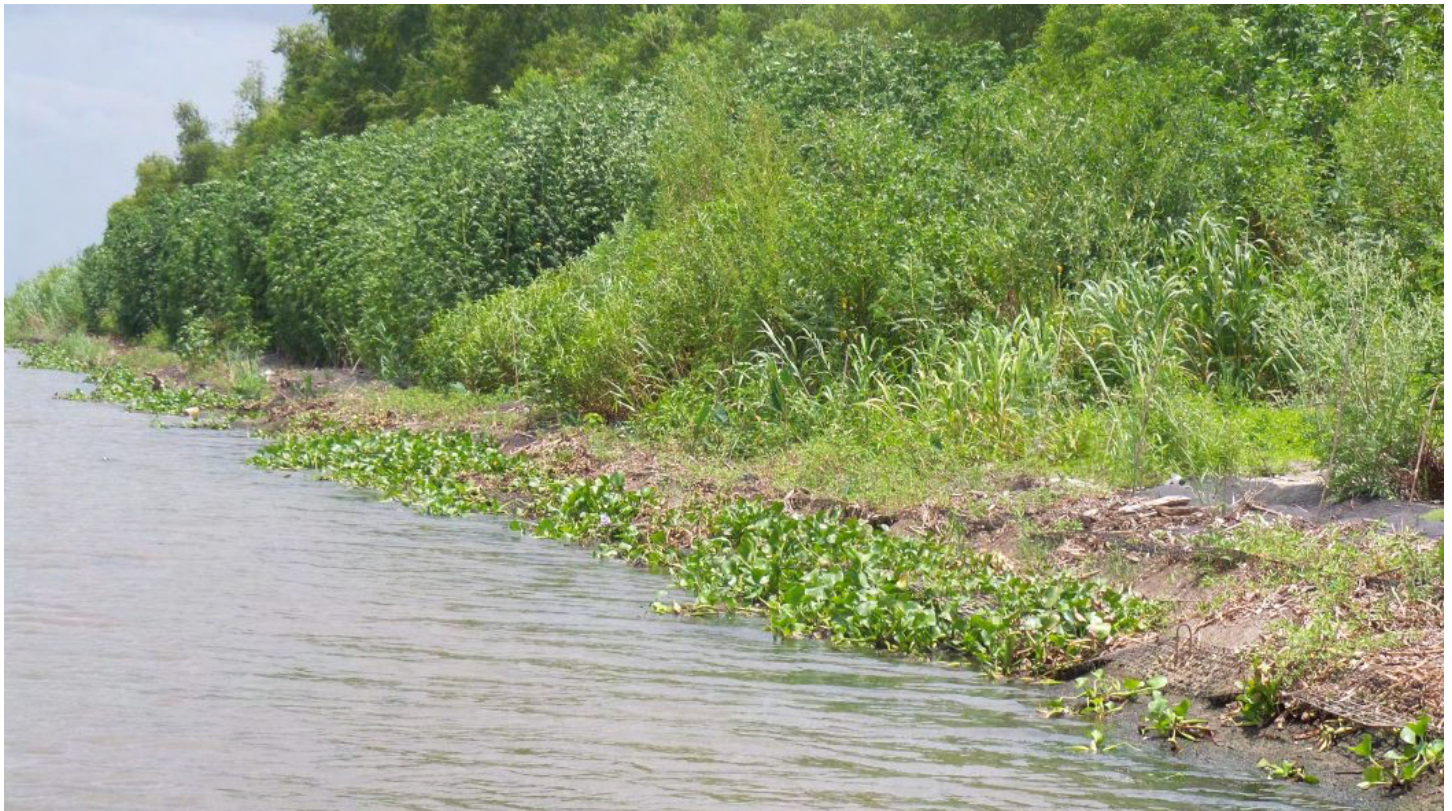
Six months after installation of EcoShield. Courtesy America’s WETLAND Foundation.
