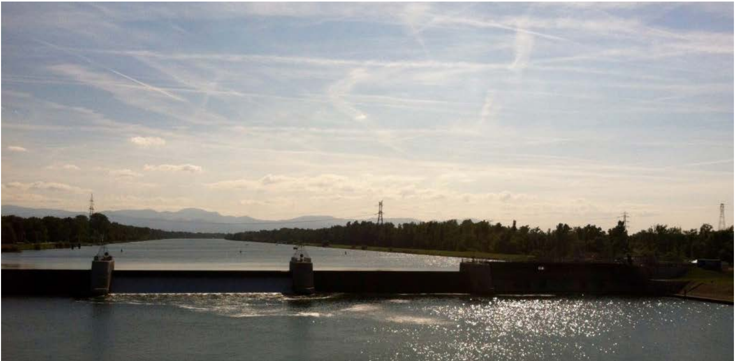
Weir dam and lock on the Rhine River at Breisach, Germany. Image courtesy of Kristen Anderson.
