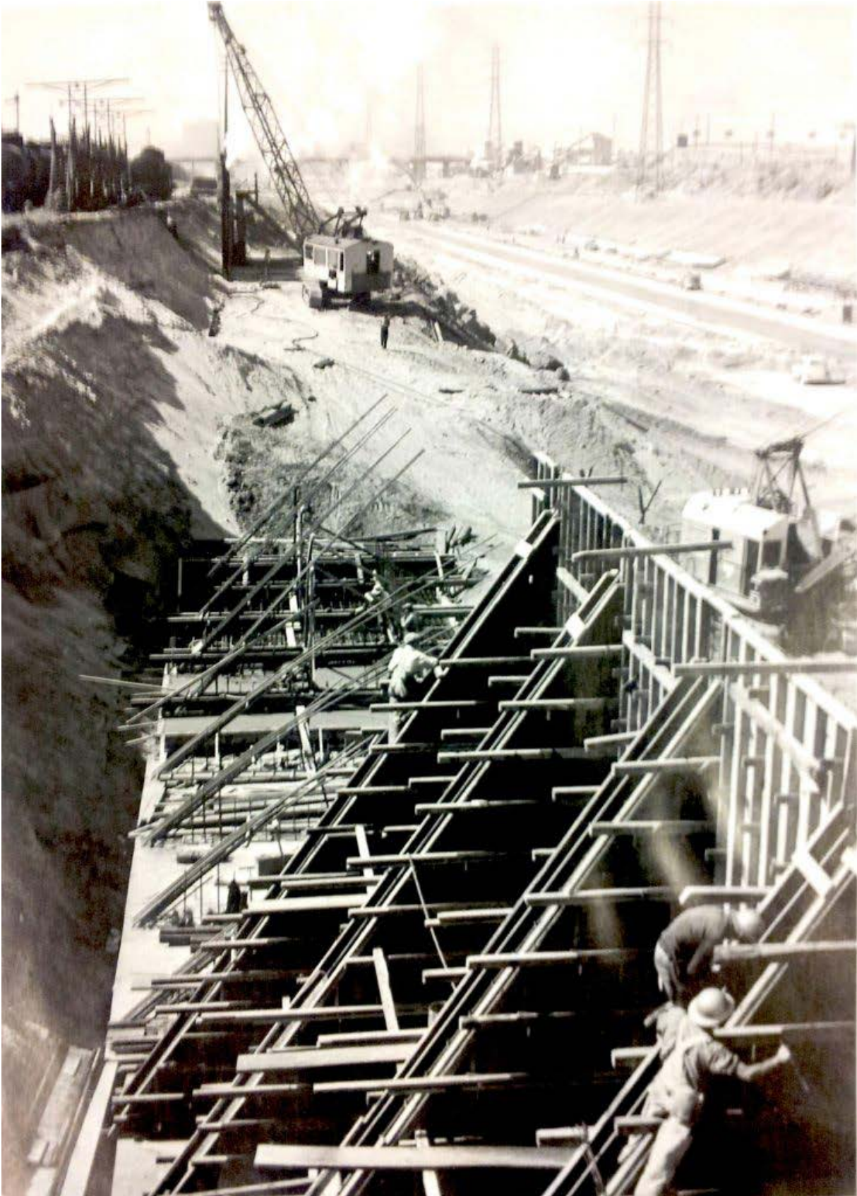
Upstream view of the Los Angeles River channel above Butte Street Bridge during construction. Image via U.S. Army Corps of Engineers Los Angeles District.
