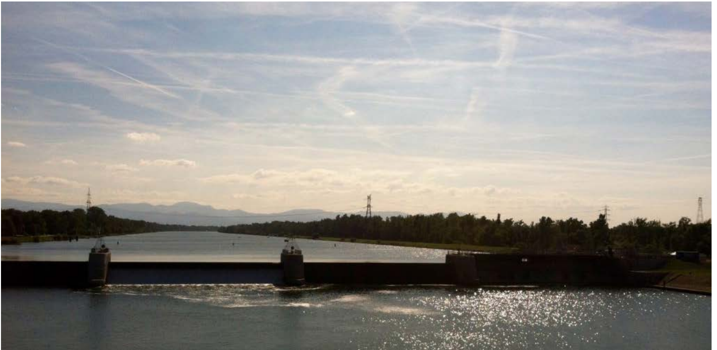
Weir dam and lock on the Rhine River at Breisach, Germany. Image courtesy of Kristen Anderson.
