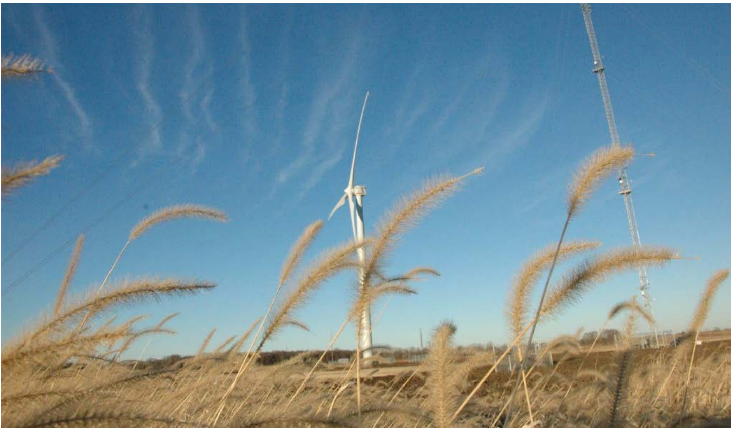
The Eolos Wind Energy Field Station consists of a fully instrumented 2.5 MW Clipper Liberty wind turbine and 400-ft meteorological tower located in Rosemount, Minnesota.
