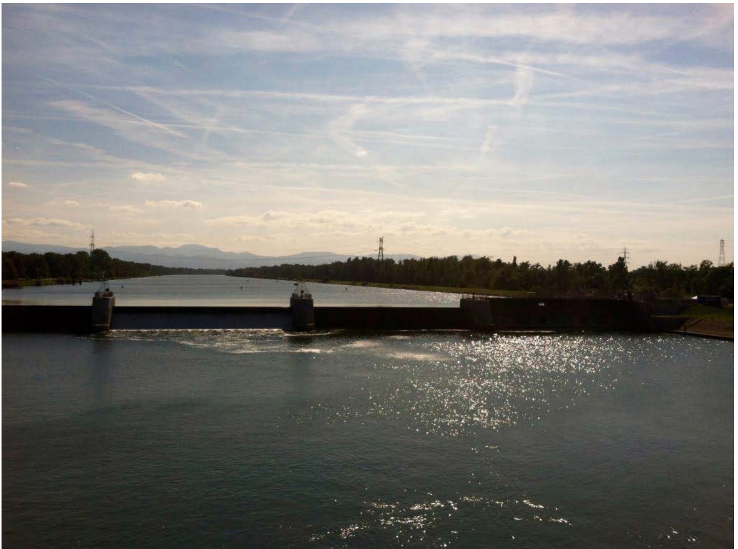
Weir dam and lock on the Rhine River at Breisach, Germany. Image courtesy of Kristen Anderson.
