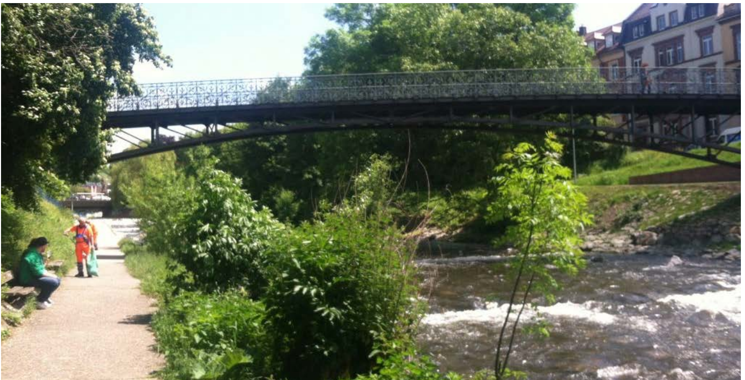
Pedestrian paths and bridges along the urban Dreisam River in Freiburg, Germany. Image courtesy of Kristen Anderson.
