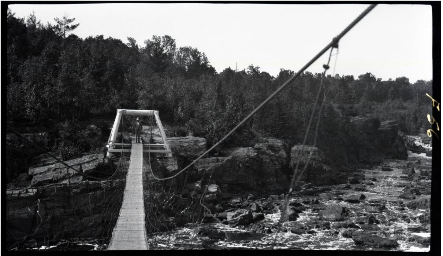
Jay Cooke State Park Suspension Bridge, 1929. Image courtesy of University of Minnesota Duluth, Kathryn A. Martin Library, Northeast Minnesota Historical Center Collections.
