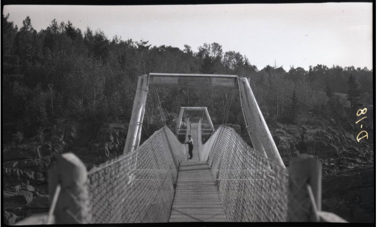
Jay Cooke State Park Suspension Bridge, 1929.
