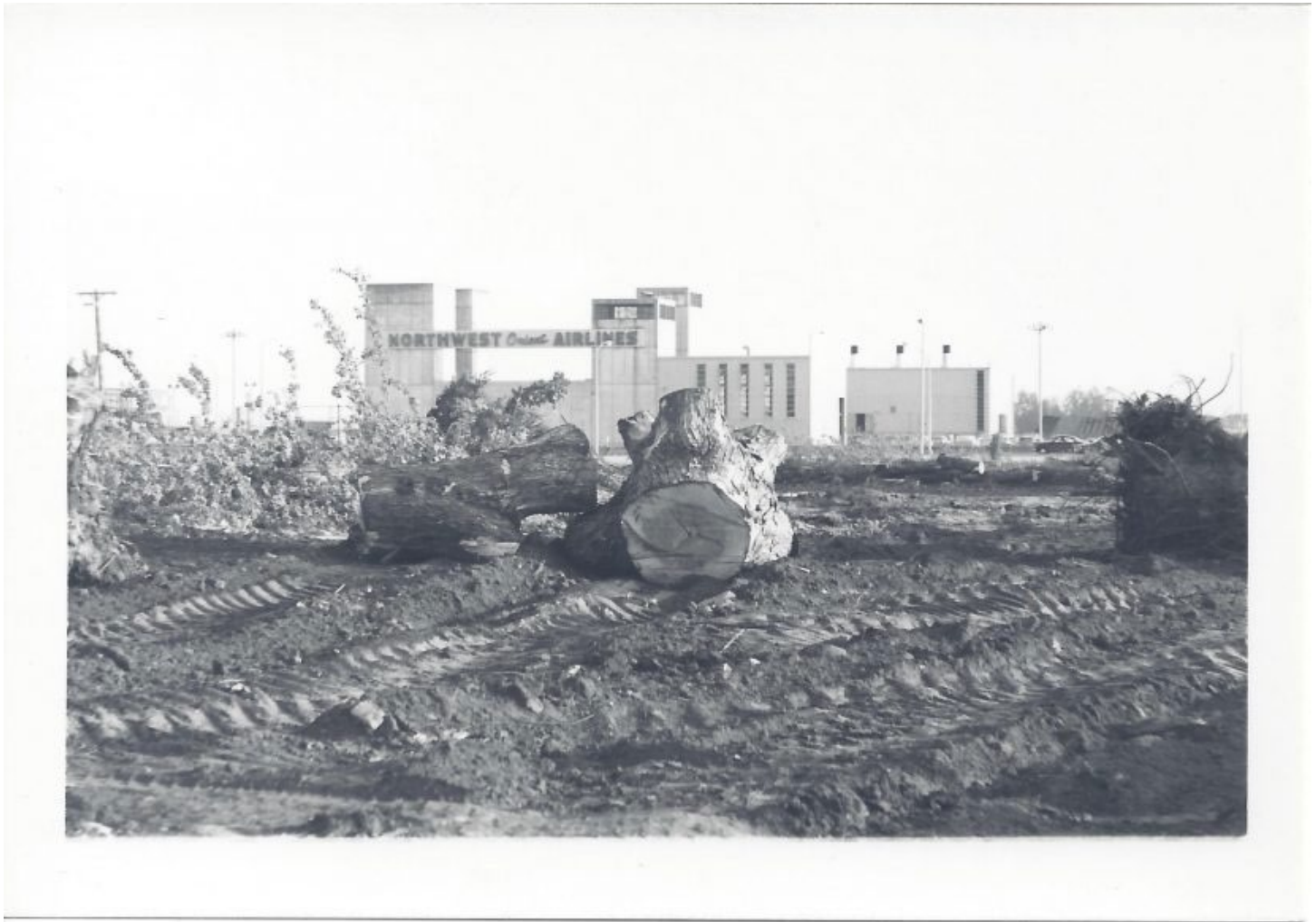
Demolition for airport construction. Image by Richard E. Watson, M.D., courtesy of the author.
