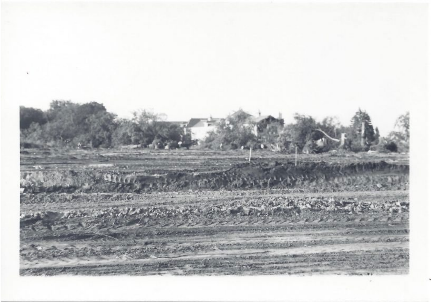
Officers Row demolished for airport construction. Image by Richard E. Watson, M.D., courtesy of the author.
