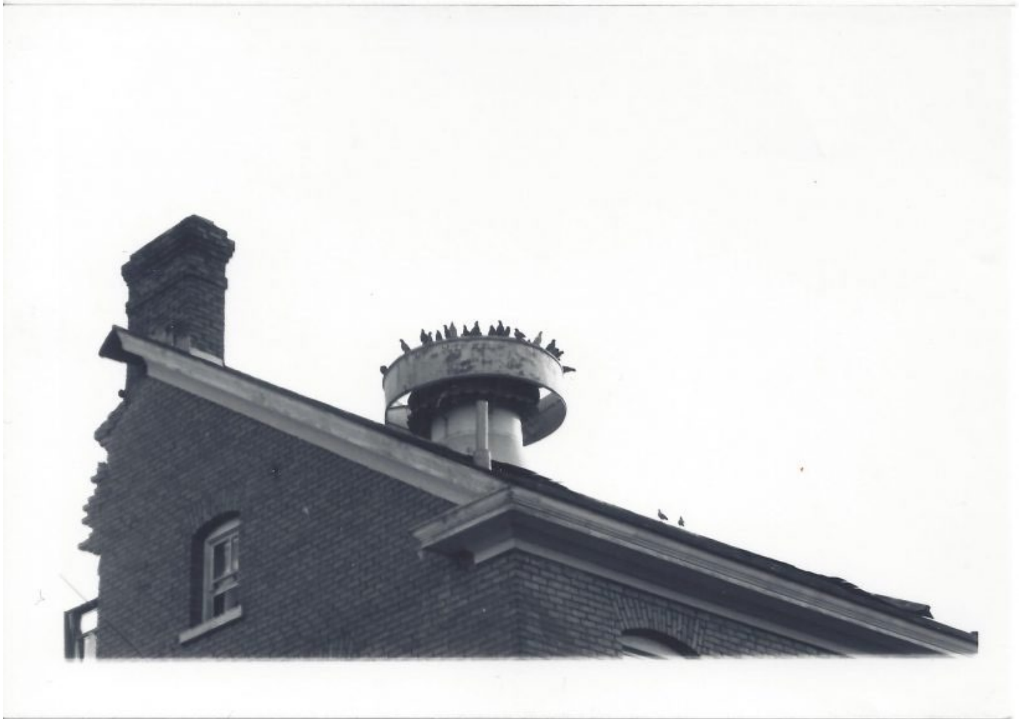
Barracks buildings on Taylor Avenue being torn down. Image by Richard E. Watson, M.D., courtesy of the author.
