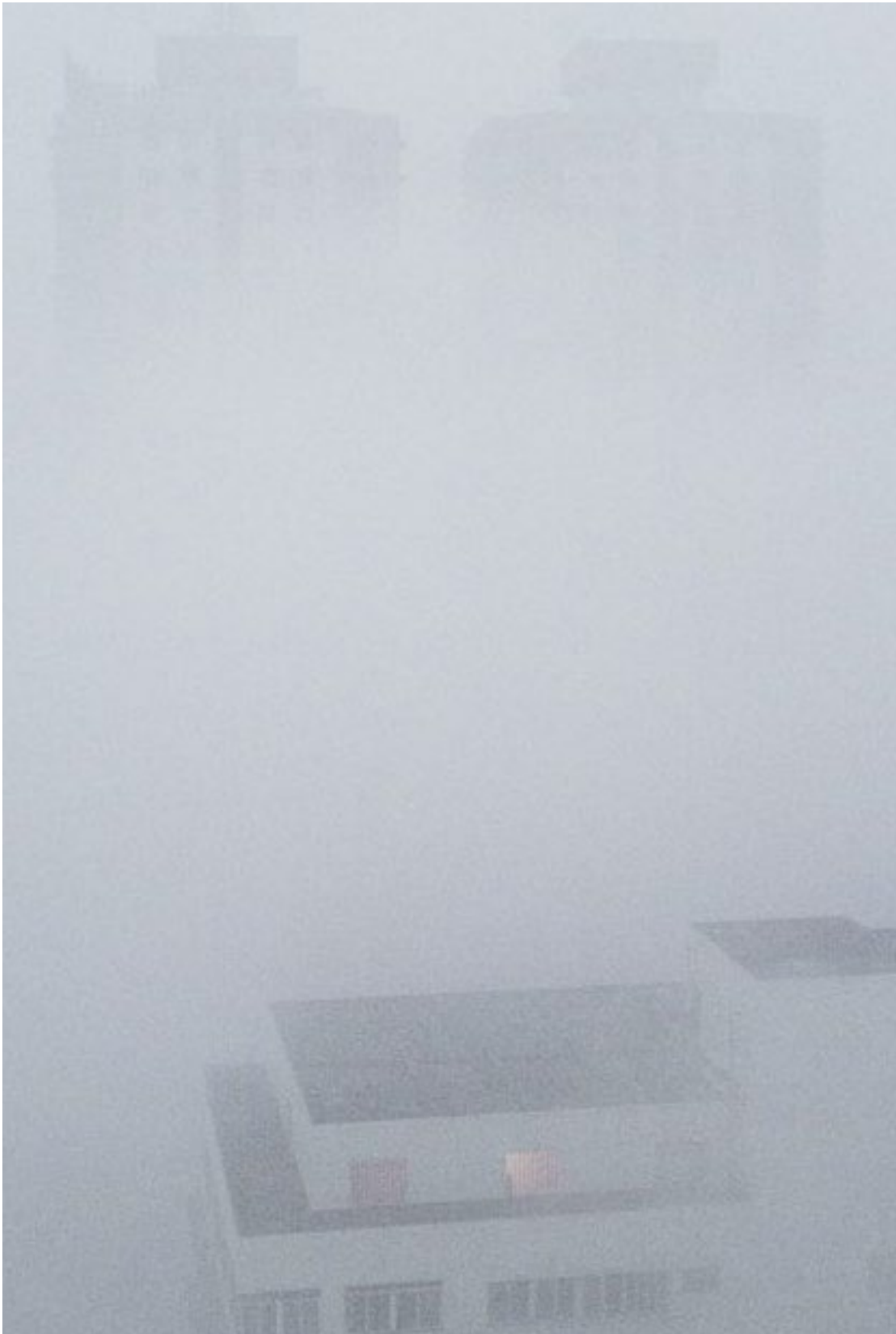
New construction higher up on the hills of the Yangtze River. Chongqing, China. 2000.
