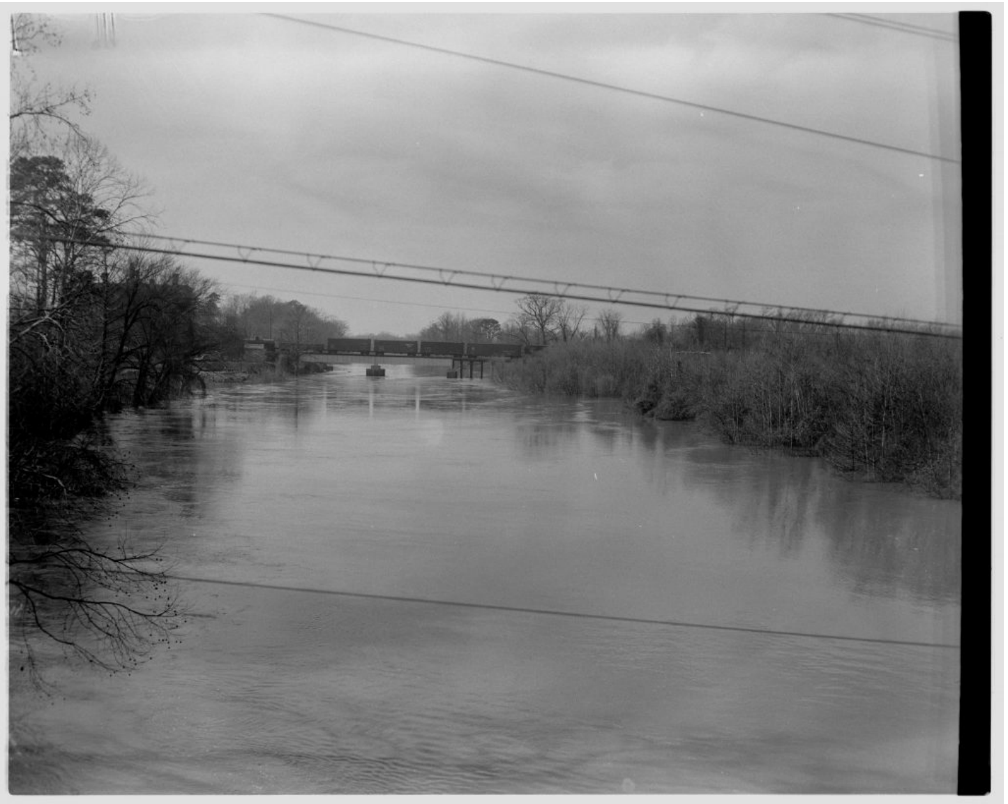
Tar River water level elevated almost to reach the bridge. Date from negative sleeve. Daily Reflector (Greenville, N.C.), January 26, 1954.
