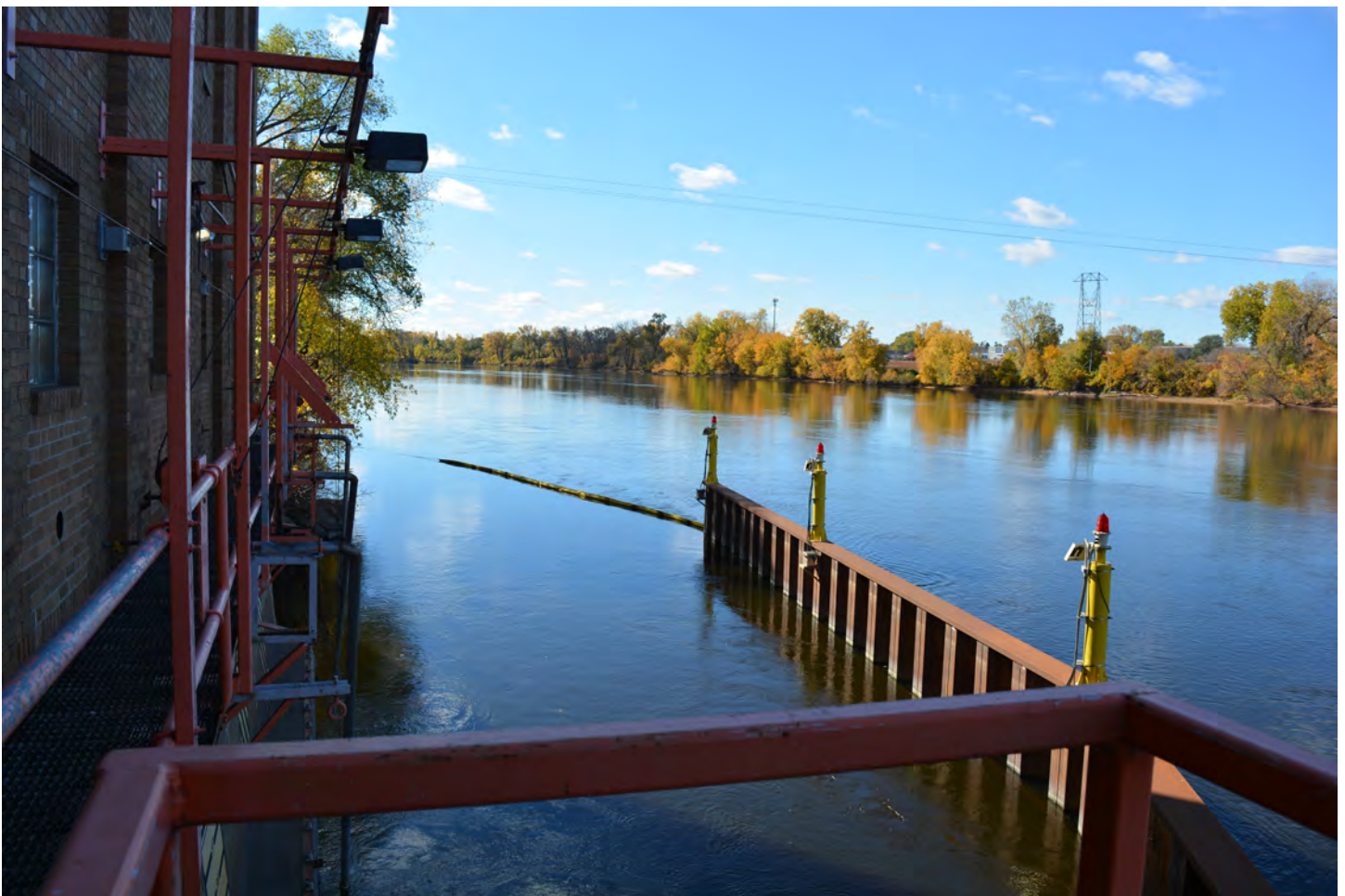
Drinking water intake for the City of Minneapolis.
