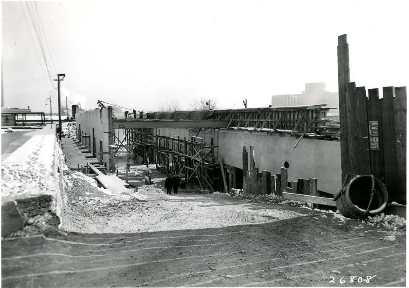
1937 construction of the model floor, SAFL's largest modeling/experimental space with access to the adjacent supply channel (middle of photo). Note the NSP (Northern States Power) diversion canal to the north (left of picture).
