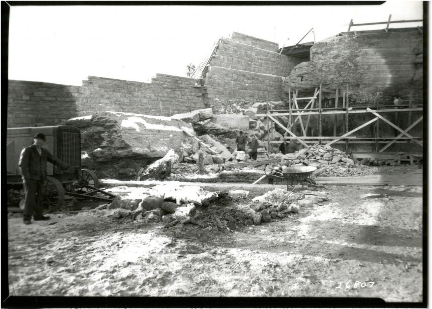
SAFL's exterior walls were constructed using limestone quarried on site, 1936-37.
