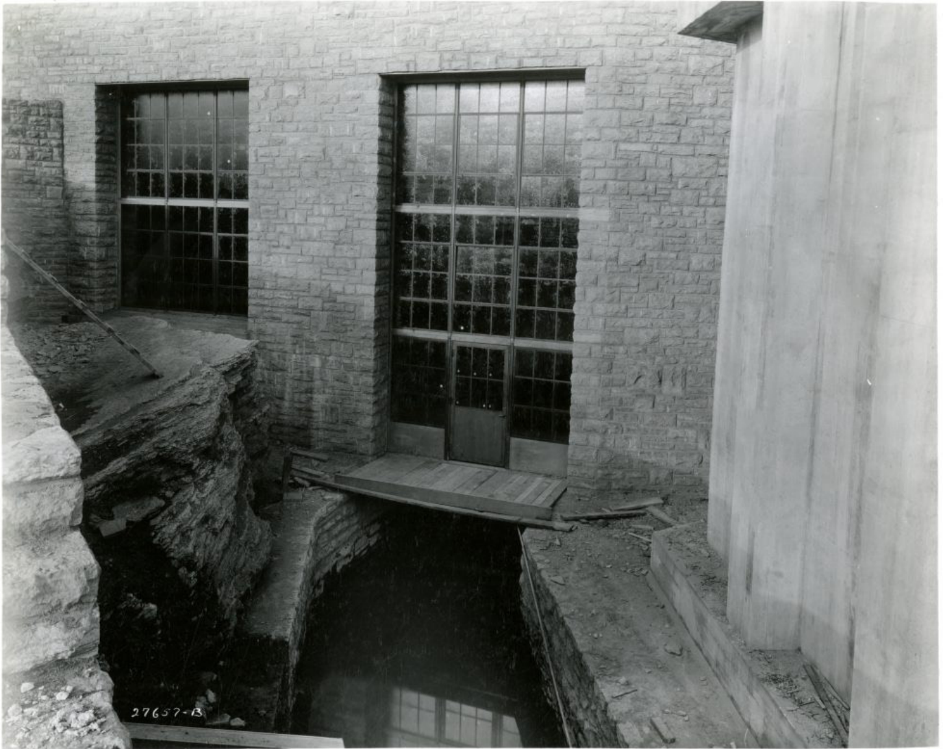
The basement level of the laboratory is constructed over the top of the outflow channel where water exits the building and rejoins the Mississippi River below the falls.
