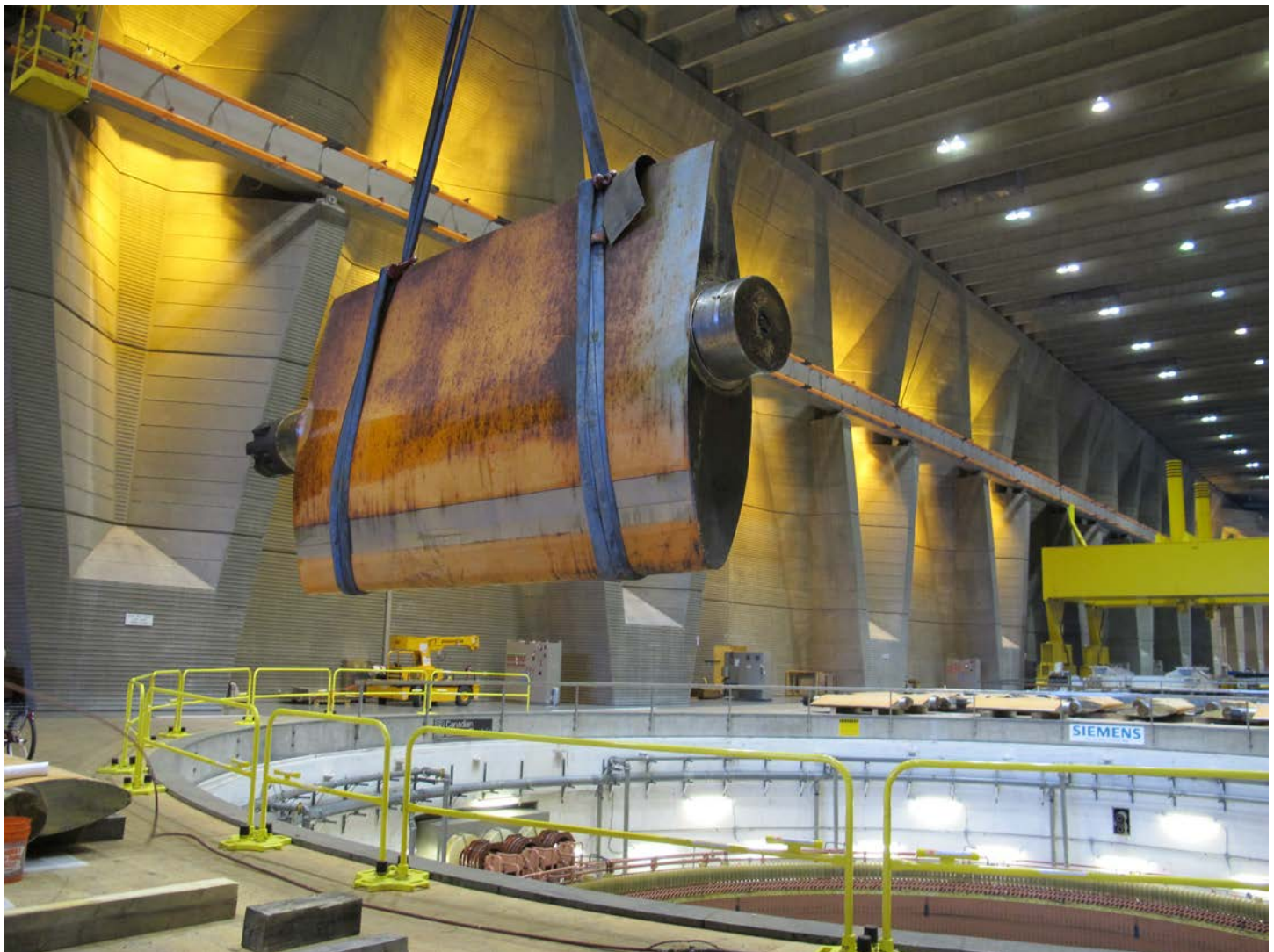
This wicket gate removal at the Grand Coulee Dam on the Columbia River illustrates the massive scale of our water infrastructure. Image courtesy of Bonneville Power Administration.
