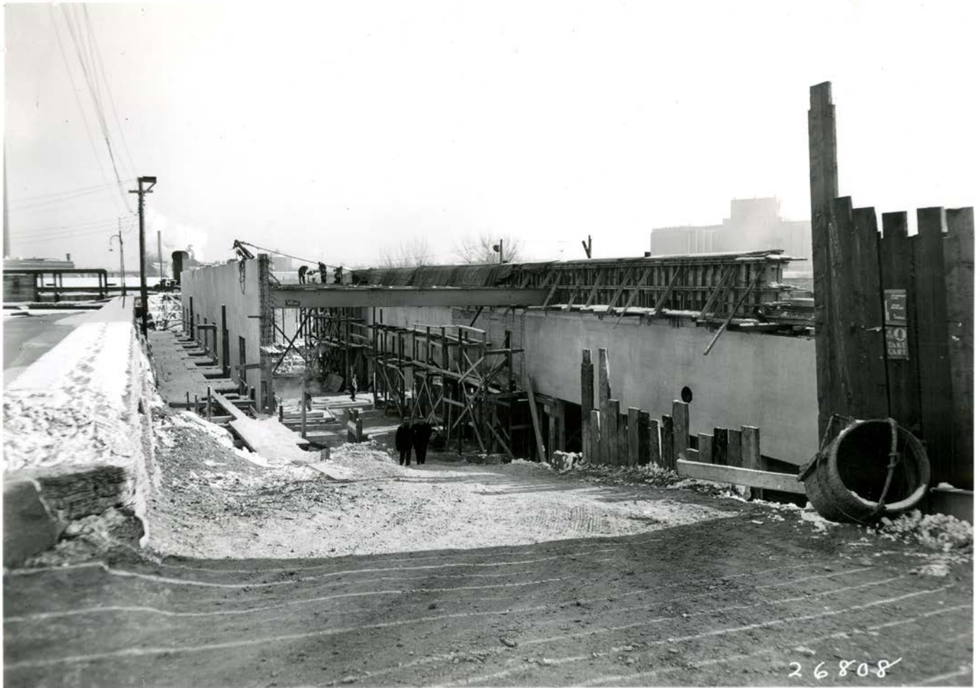
1937 construction of the model floor, SAFL's largest modeling/experimental space with access to the adjacent supply channel (middle of photo). Note the NSP (Northern States Power) diversion canal to the north (left of picture).
