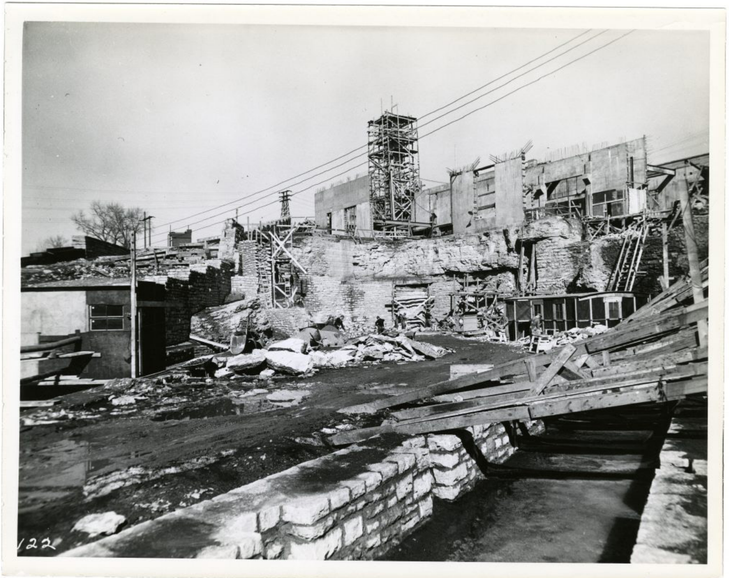
Laboratory construction in 1936 included excavation of approximately 30,000 lbs of limestone to expand the bottom floor where SAFL's outflow channel takes diverted water back to the river below St. Anthony Falls.
