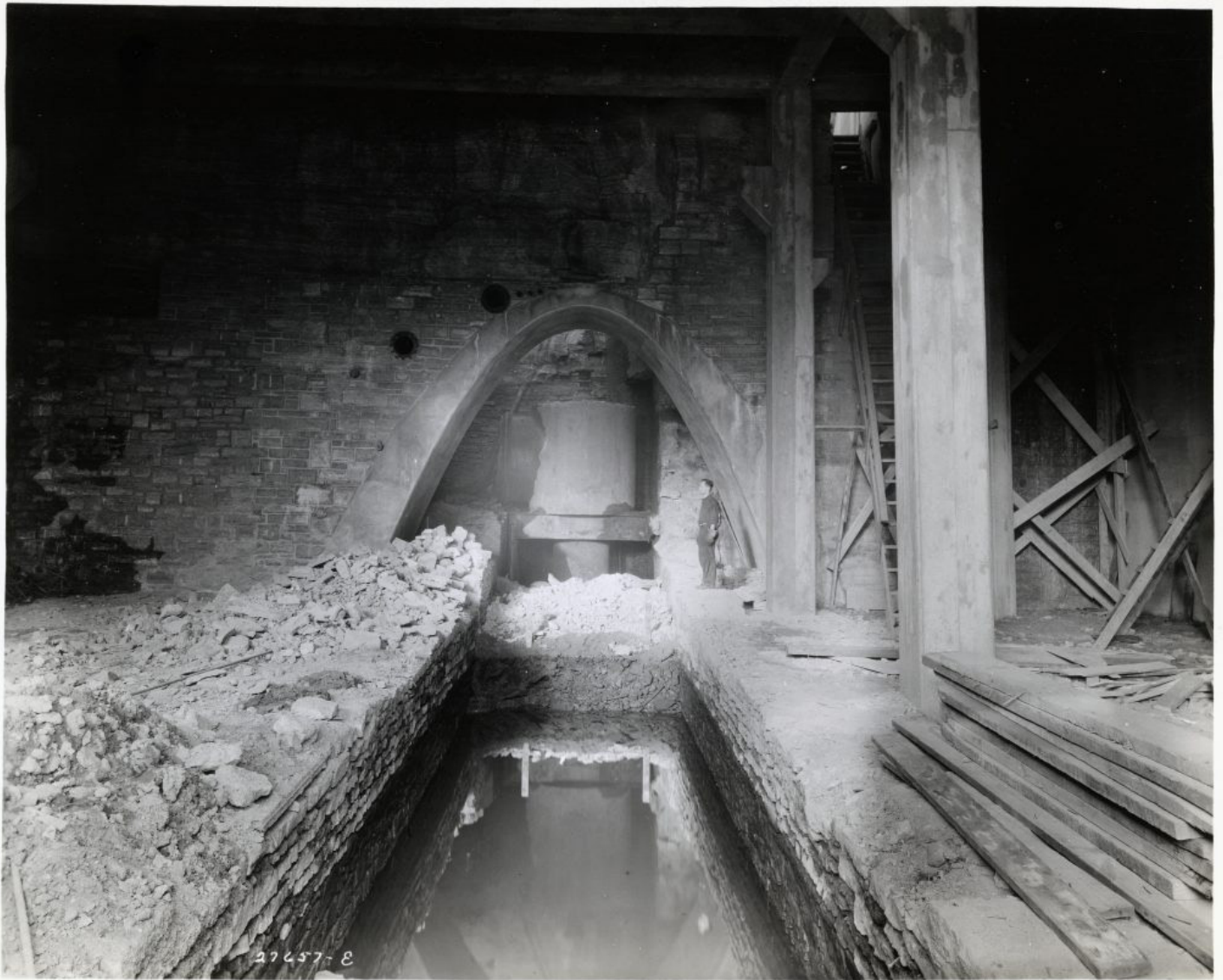
The original outflow channel that moves water from the laboratory back to the Mississippi River was constructed for the former Minneapolis pumping station in the 1880s. The pumping station was demolished to make way for the lab. Note that the pumping station turbine (center of photo) still remains.
