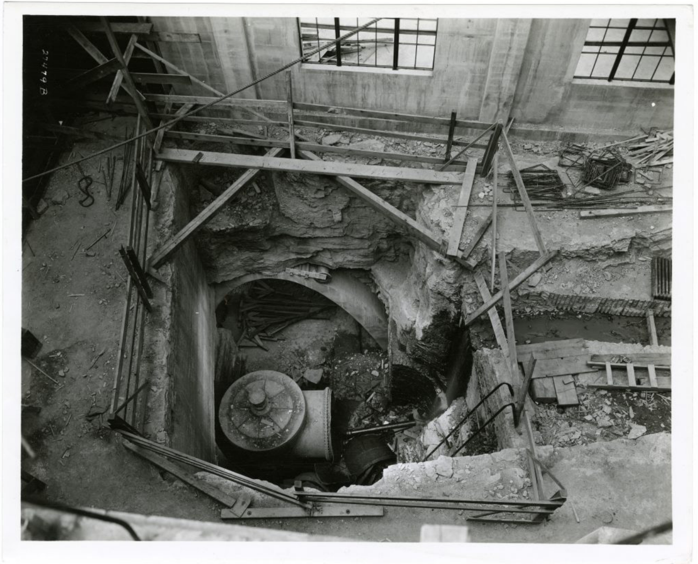
A 1936 view to the bottom of the laboratory where the turbine of the former pumping station still resided at time of construction. To this day, the basement floor of the lab is referred to as “the turbine level.”
