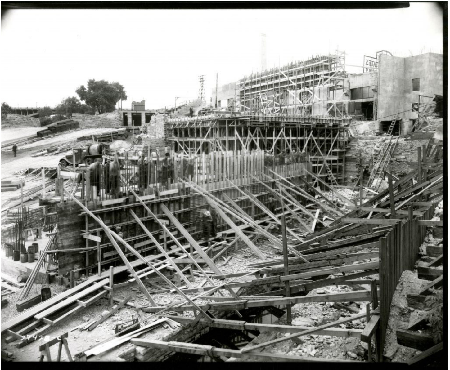
Construction photo of SAFL in 1937, showing extensive timber framing and the outflow channel, used to send water back to the river after its use in the laboratory. Viewed from near the river's edge.
