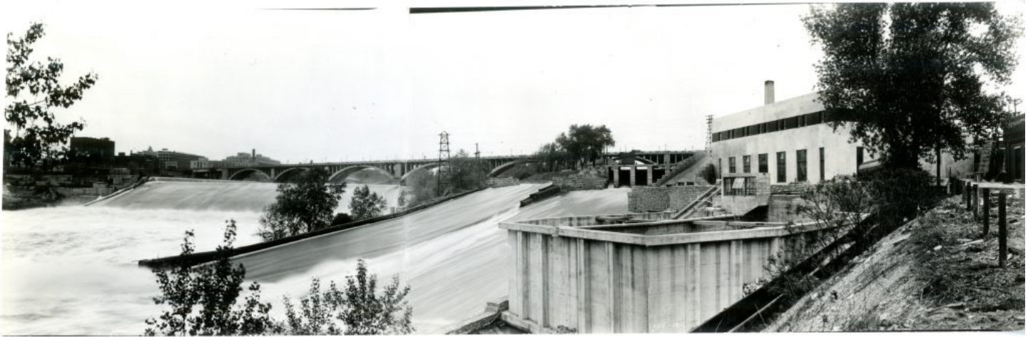
View of the St. Anthony Falls and flood bypass channel alongside the newly completed St. Anthony Falls Laboratory with the volumetric basins visible in the foreground.
