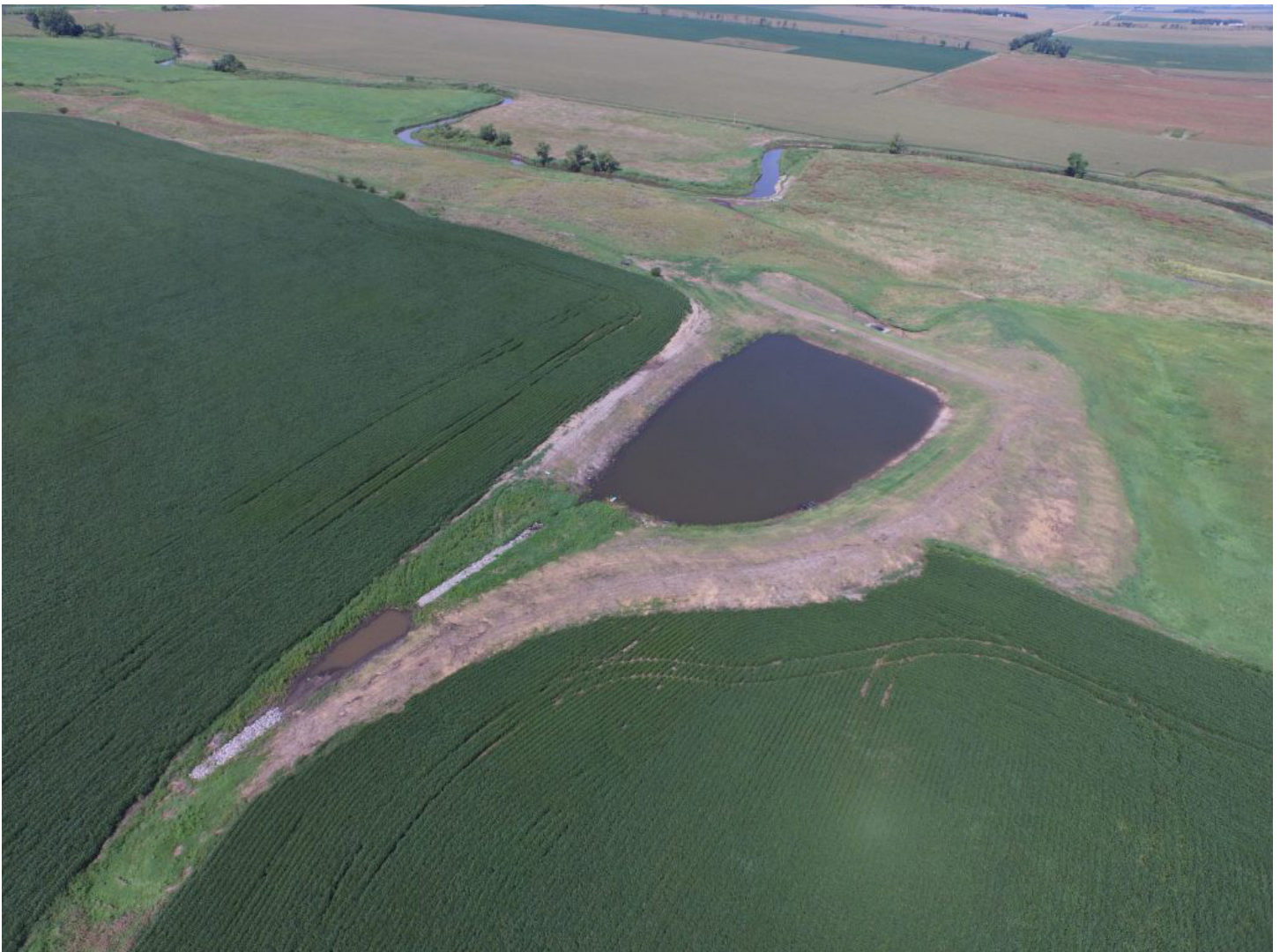
A storage pond on a western Minnesota farm collects tile runoff in the spring to be used for supplemental irrigation during summer dry spells. Image courtesy of Jake Hicks.
