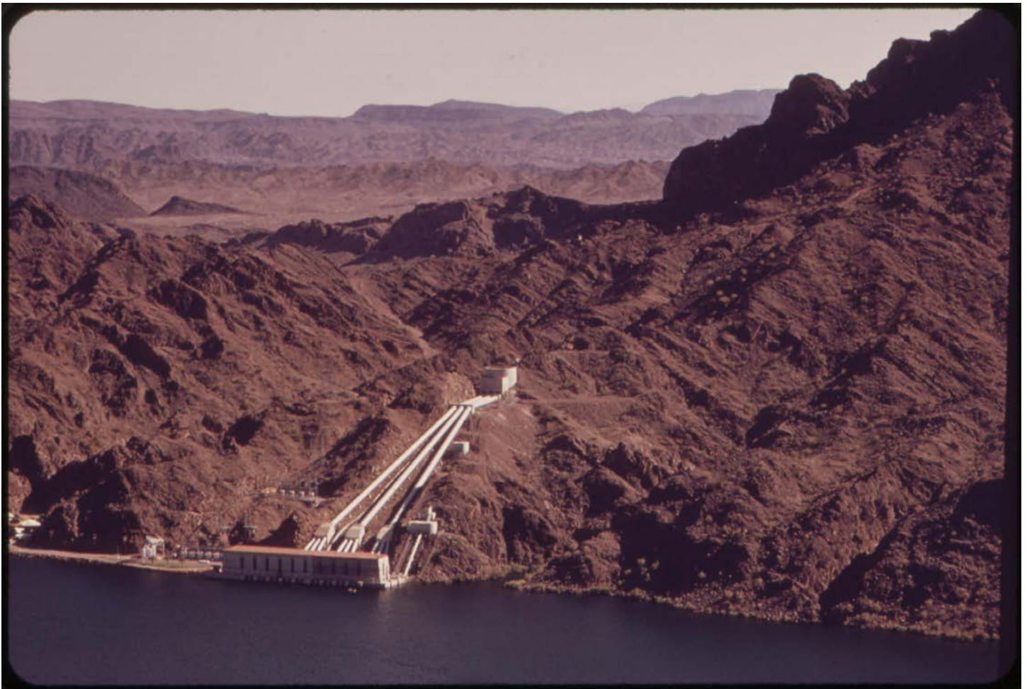
Whitsett Pumping Plant on Lake Havasu lifts the water 291 feet (89 m) for the Colorado River Aqueduct, bring water to Los Angeles. Photographer Charles O'Rear, 1972.
