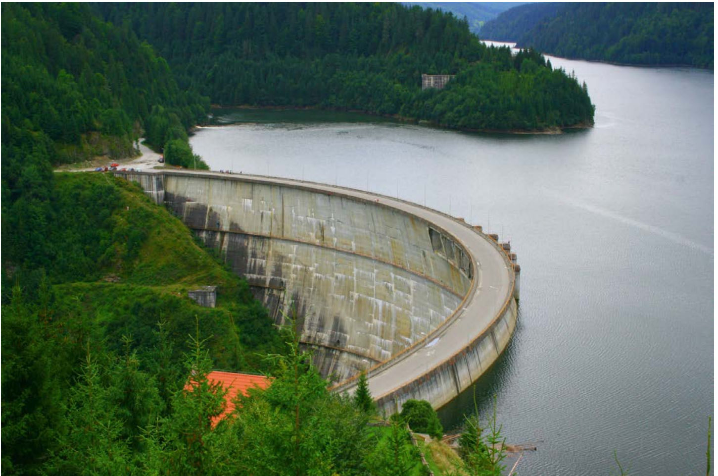
Dragan Dam in Romania. Photographer Colin Woodcock.
