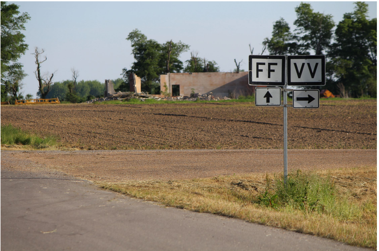
Ruins of Pinhook Union Baptist Church circa 2014. Like all buildings in the village, the church was completely submerged for more than two weeks. It was set ablaze by an arsonist soon after the water subsided and was later demolished along with remaining town buildings in 2015.
