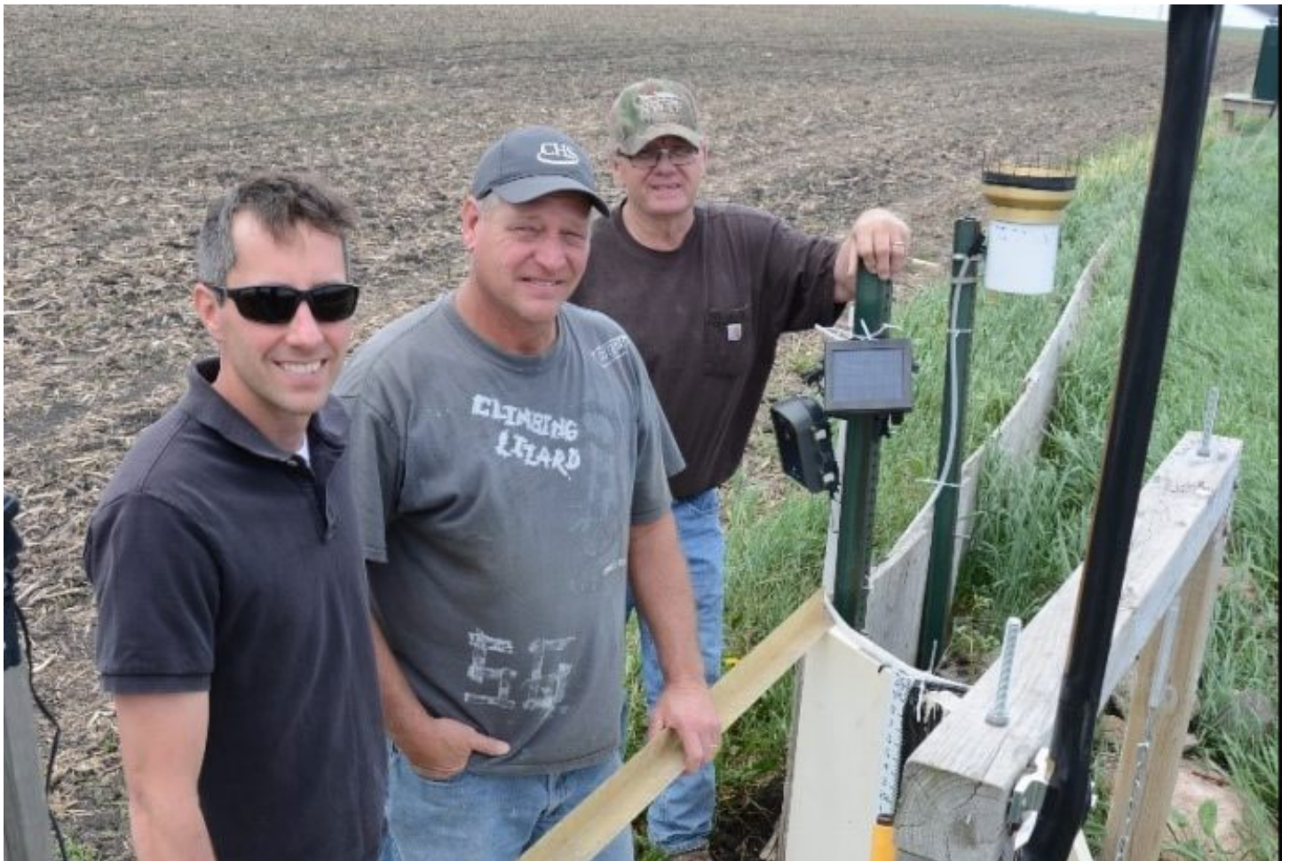
Kevin Kuehner, MDA hydrologist and researcher (left), Wayne DeWall, participating farmer (center), and RRFSP walkover technician Ron Meiners (right) pause at the edge-of-field monitoring station in DeWall's field. Data collected at this station over many years is now informing on-farm management decisions throughout the region. Image courtesy of Paula Mohr, "The Farmer" magazine.
