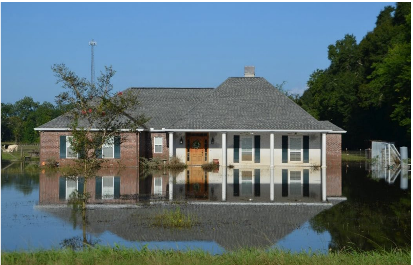
Figure 4. Slab-on-grade house that flooded, Ascension Parish. August 2016. Image courtesy of the author.
