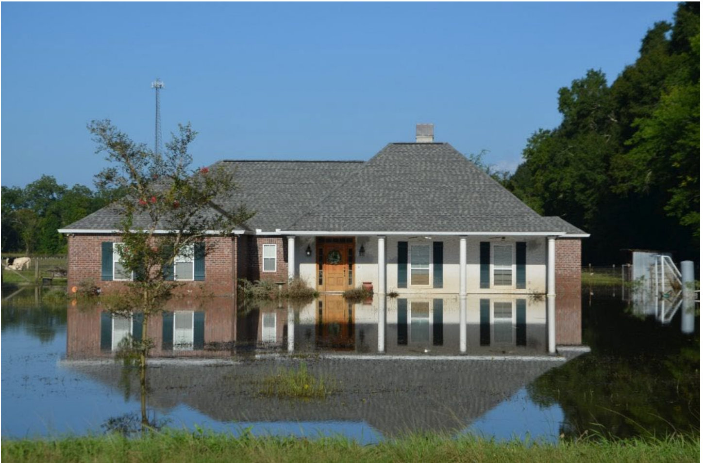
Slab-on-grade house that flooded, Ascension Parish. August 2016. Image courtesy of the author.
