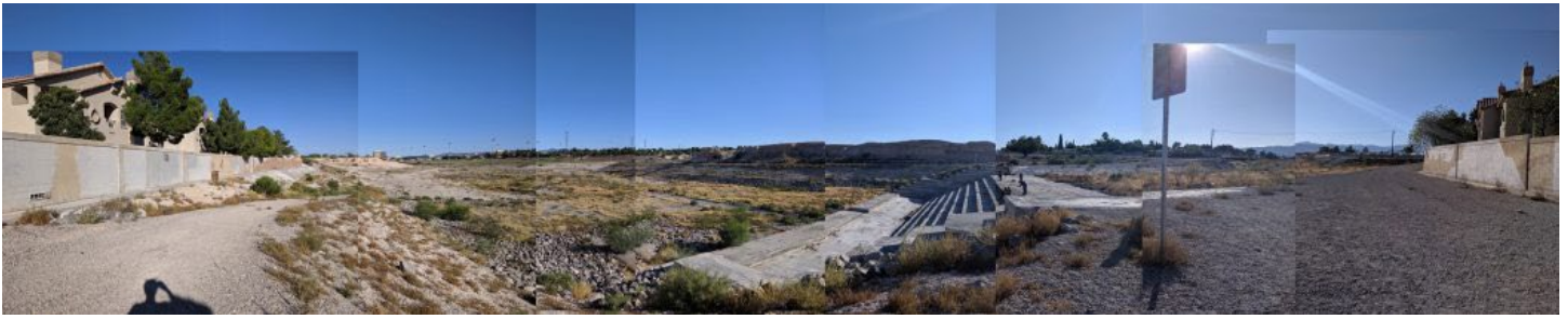
The inlet of the Tropicana Detention Basin, where a public park sits within a piece of flood control infrastructure. Image courtesy of the author.
