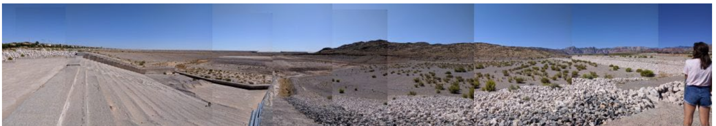
Red Rock Detention Basin at the northwest of Las Vegas, which intercepts flood water coming off of La Madre Mountains and Red Rock Canyon National Conservation Area.
