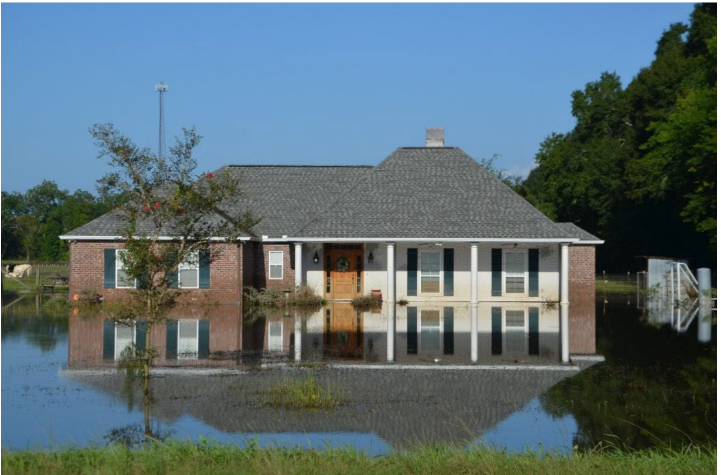
Slab-on-grade house that flooded, Ascension Parish. August 2016. Image courtesy of the author.
