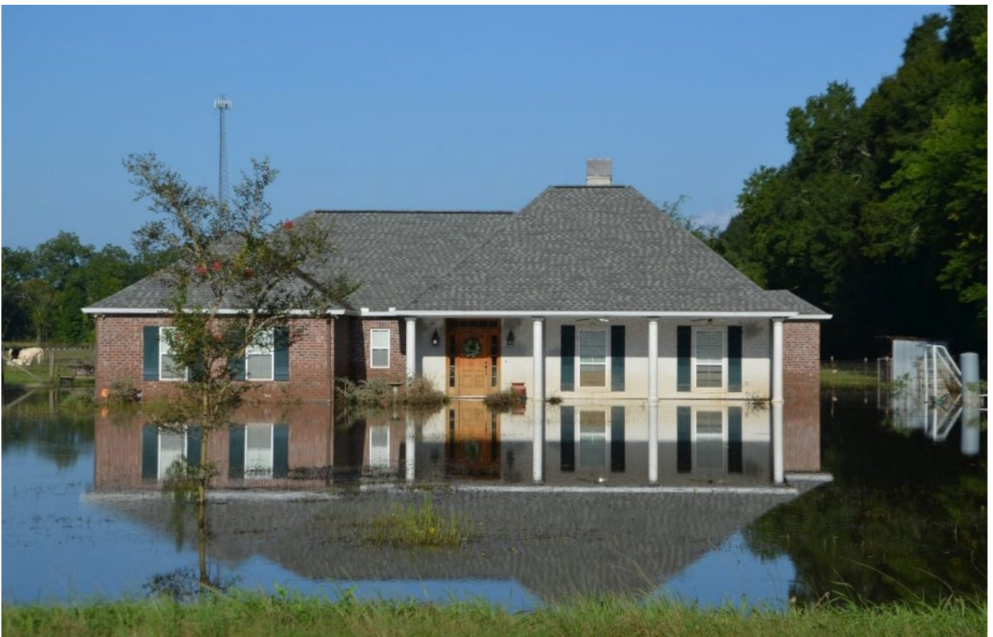
Figure 4. Slab-on-grade house that flooded, Ascension Parish. August 2016. Image courtesy of the author.
