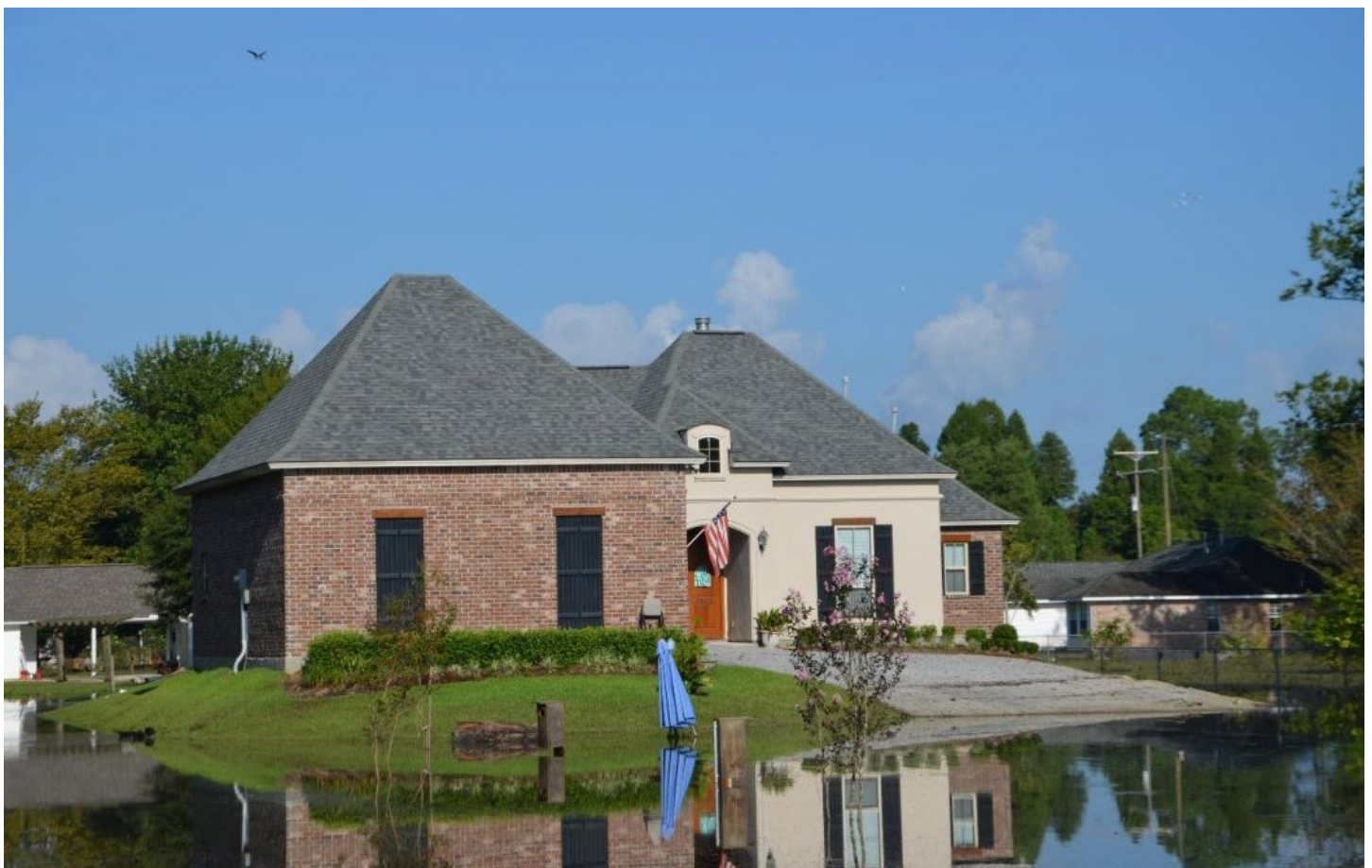
Figure 5. House constructed on fill, Ascension Parish, August 2016. Image courtesy of the author.
