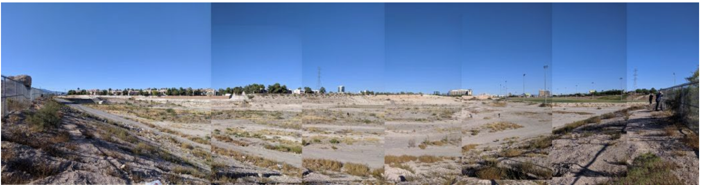
Looking into the Tropicana Detention Basin, where a public park sits within a piece of flood control infrastructure. Image courtesy of the author.
