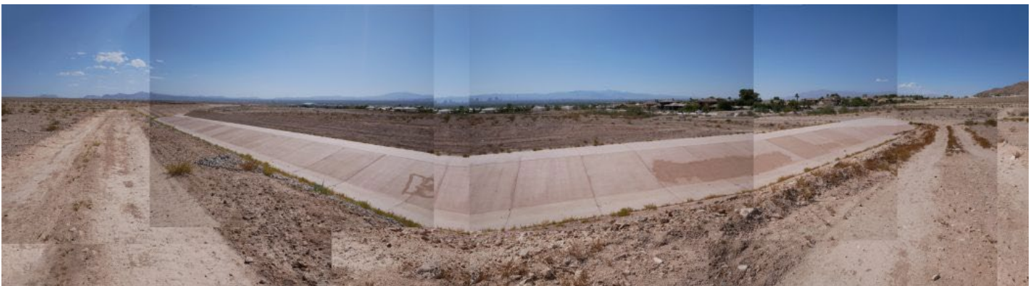
Water infrastructure at the eastern edge of Las Vegas that intercepts flood water coming off of Frenchman Mountain. Image courtesy of the author.
