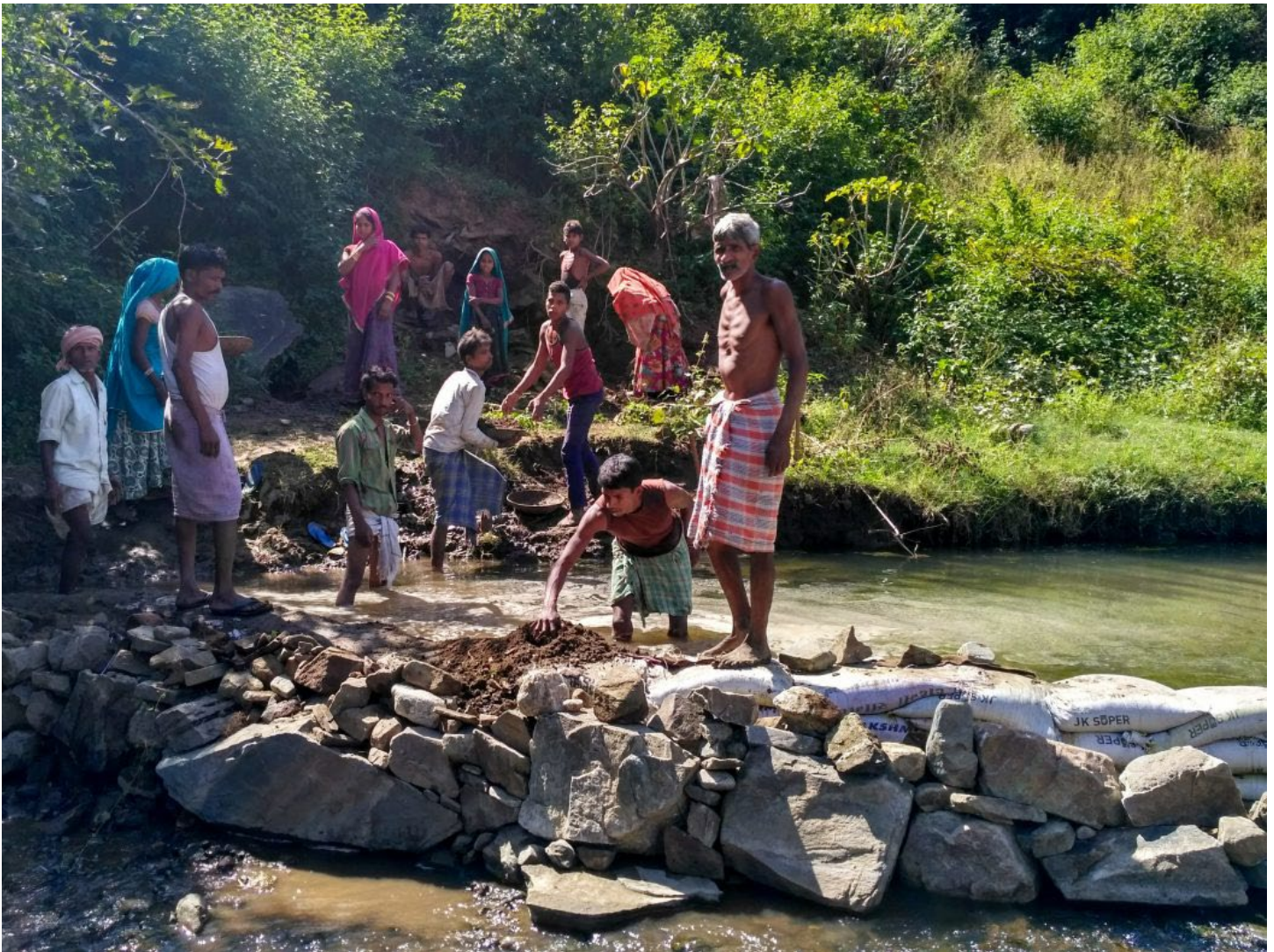
Community members participating in the construction of a boribund in Karech. Image courtesy of the author.
