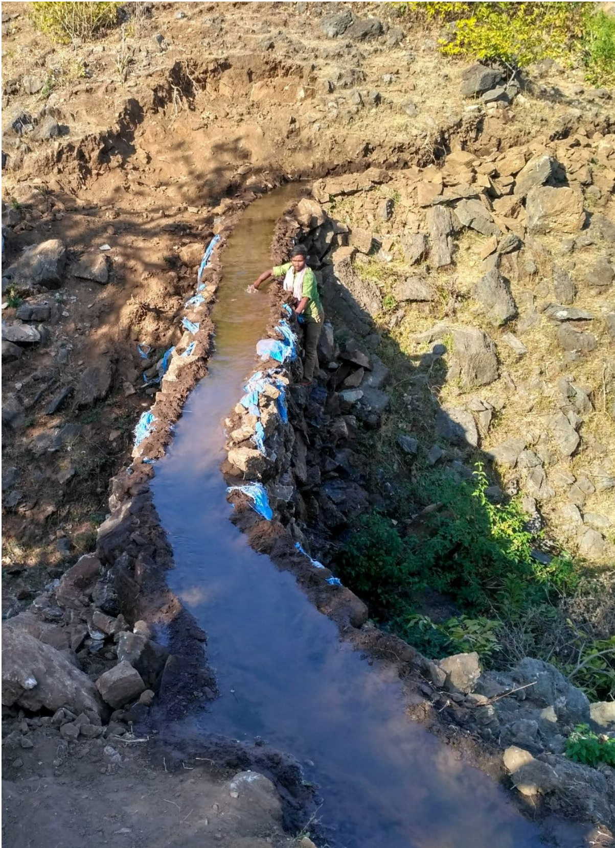
A dhora cuts across a natural drainage in Karech. Torrential rains and consequent high flow in the channels often destroy these structures and they have to be constructed again. Image courtesy of the author.
