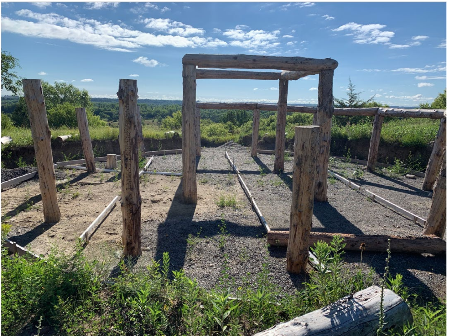
Waiting for the roof poles and Earth covering for the earthlodge at Makoče Ikikčupi. Image courtesy of Jim Rock.
