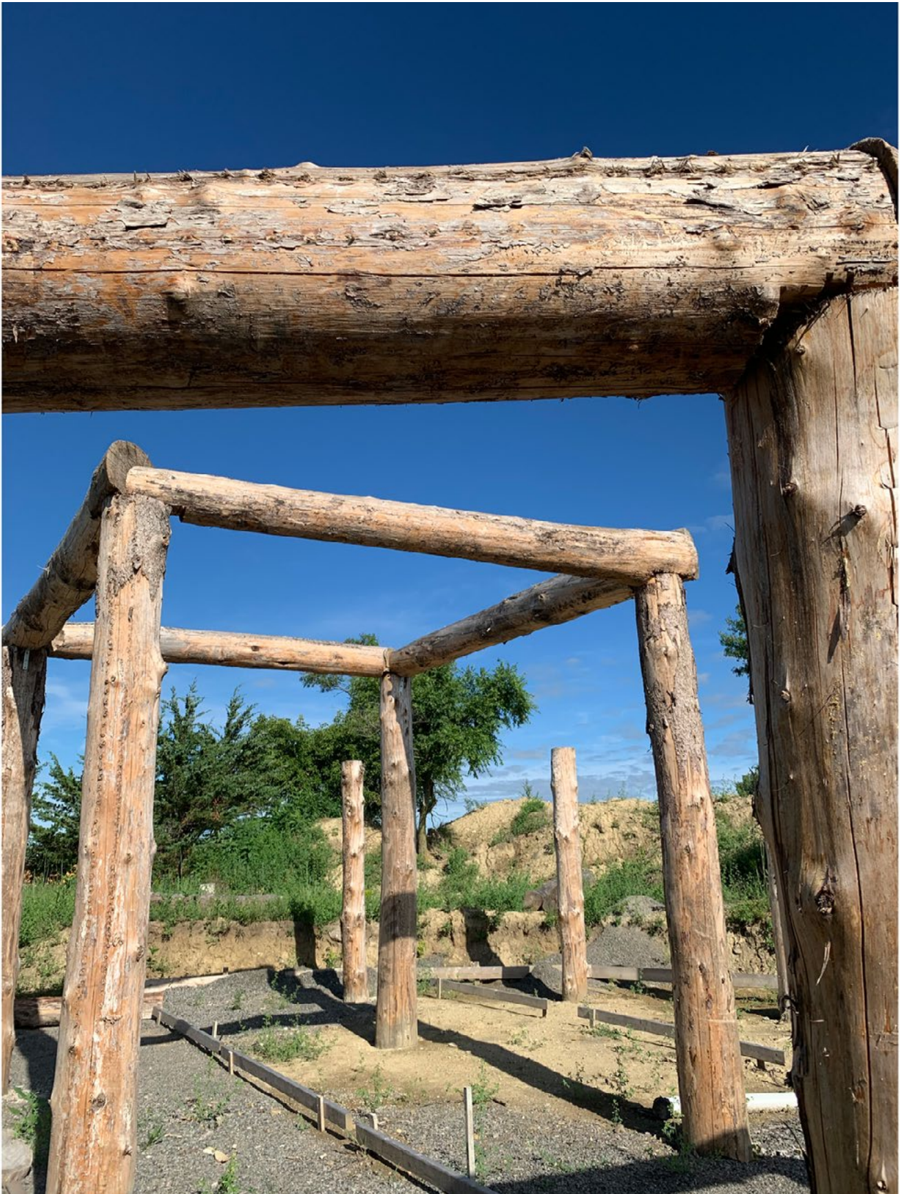
Earthlodge construction at Makoče Ikikčupi. Image courtesy of Jim Rock.
