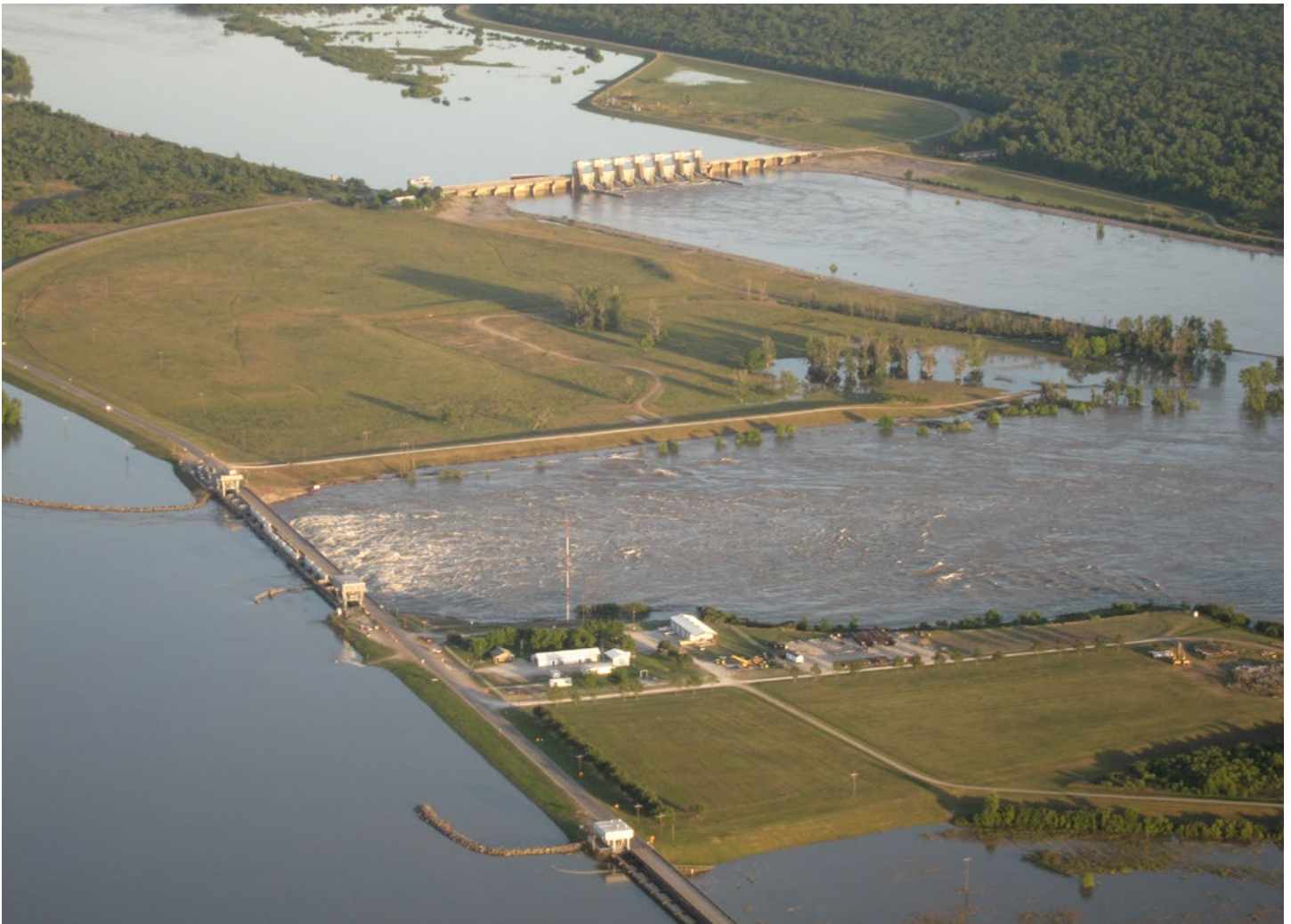
This photograph of the Old River Control Structure in Louisiana shows some of the intricate arrangement of floodgates and levees keeping each river to its course. This image was taken during the flood of 2011 and clearly shows inundation along the banks. Image by Tobin Fricke, via Flickr (CC BY-SA 2.0).
