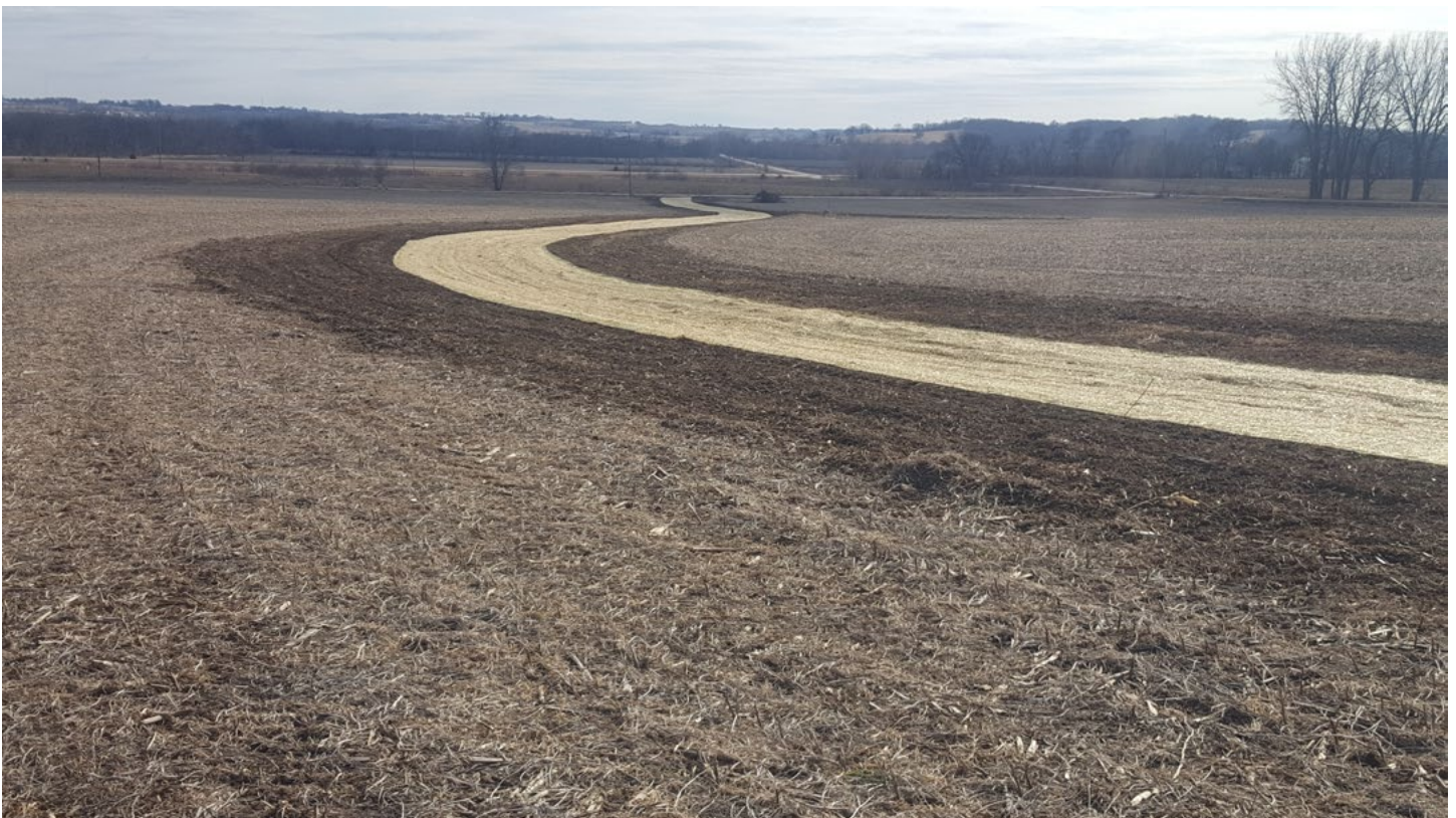
Grassed Waterway: Water needs a way to move off a farm after weather events, whether it is subsurface or above ground. Grassed waterways are purposefully shaped and planted with strong-rooted grasses to help channel water above ground. The lighter area in the photo has been shaped and planted with grass seed in straw mat to help with establishment. Image courtesy of Mollie Aronowitz.
