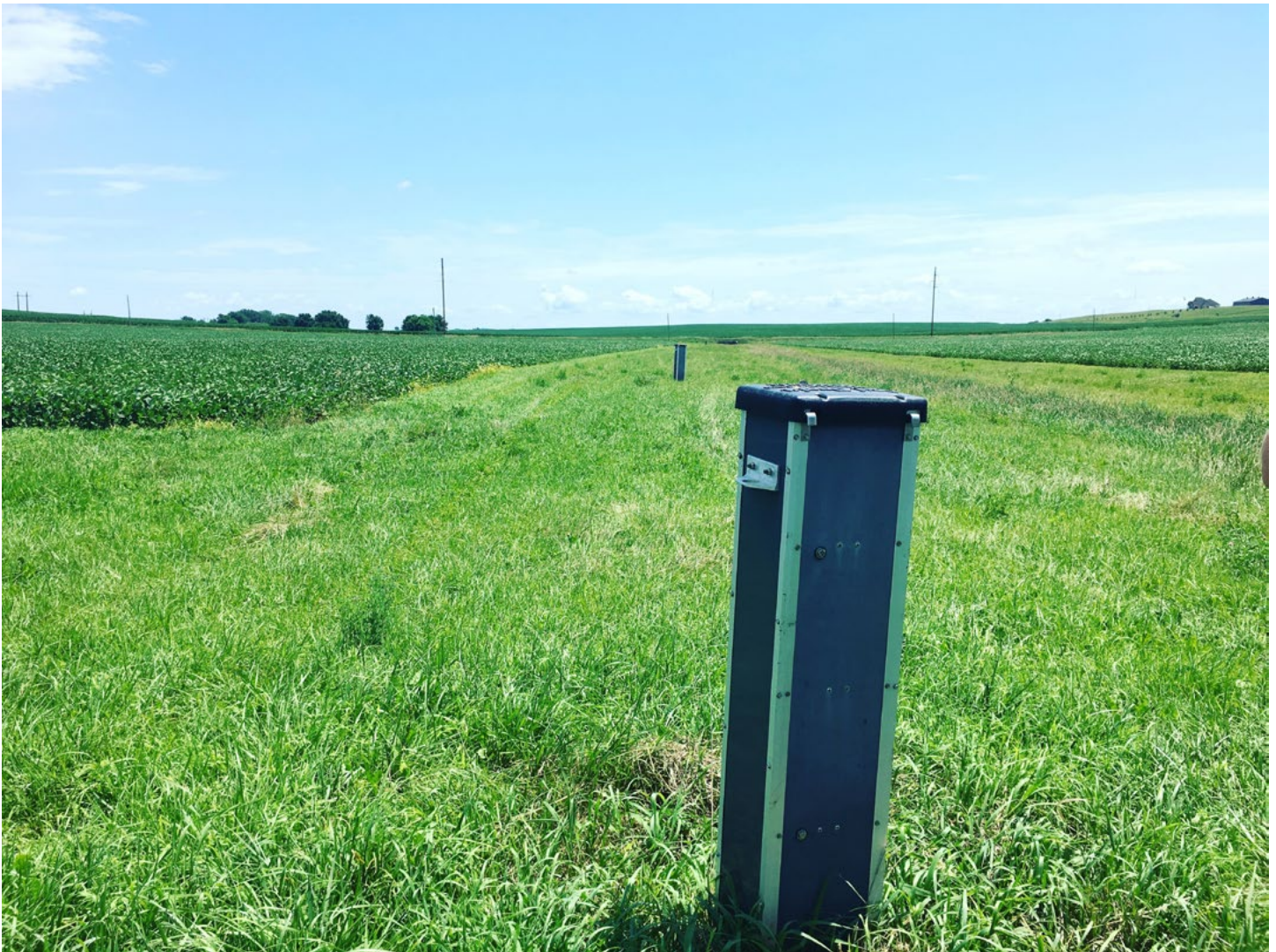
Saturated Buffers: Draining farmland with subsurface tile is critical to corn and soybean production in Iowa, and we are learning how to treat tile water before it leaves the farm. The control structures shown in the photo direct tile water to lateral lines running parallel to the drainage ditch to allow water to filter through the soil before entering the stream. When given the chance, living roots are a willing and efficient cleaner of water. Image courtesy of Mollie Aronowitz.
