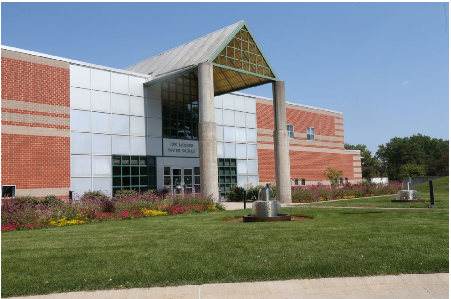
Des Moines Water Works provides safe, affordable drinking water to 600,000 central Iowans from three treatment sites, including one on the Raccoon River in Des Moines Water Works Park. Image courtesy of Des Moines Water Works.
