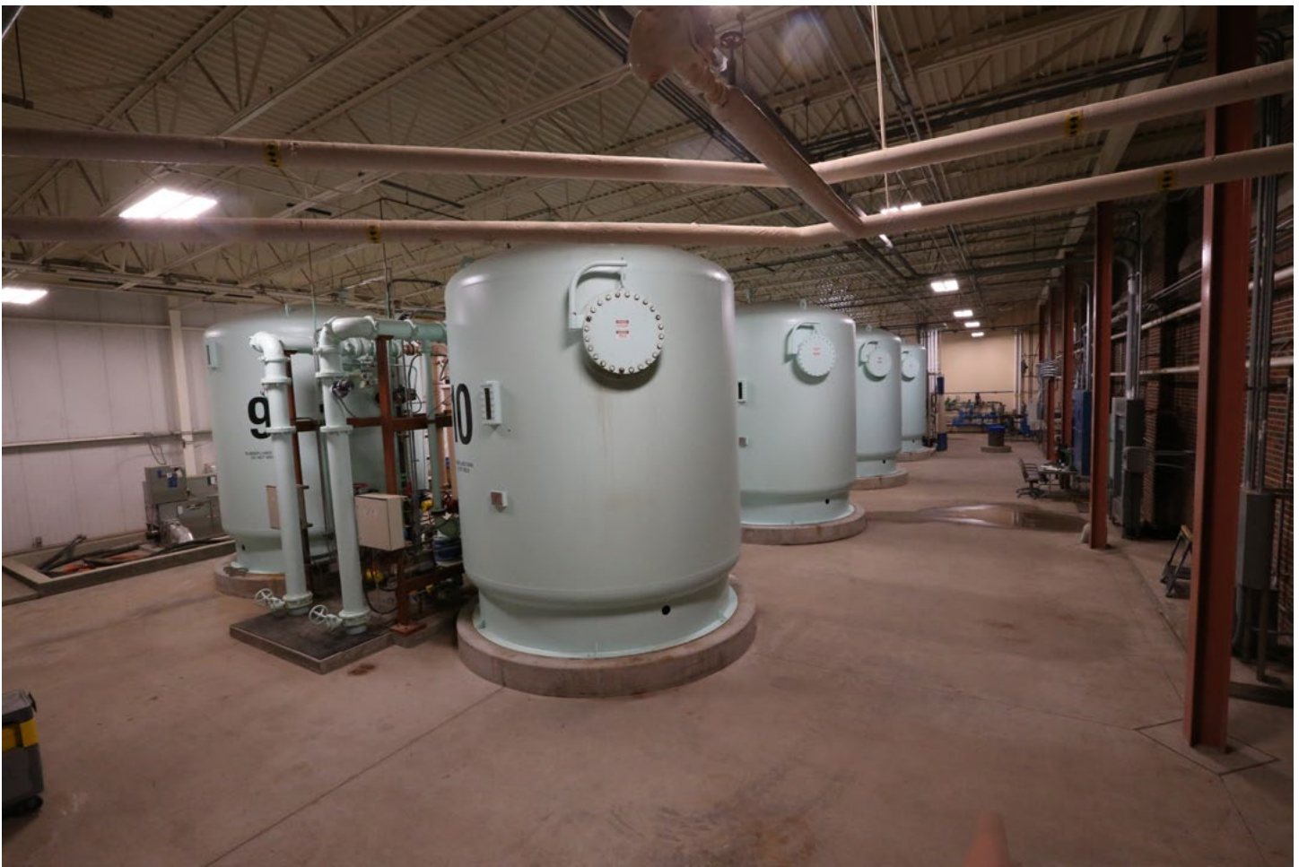
Nitrate concentrations in the Raccoon and Des Moines Rivers, two of our drinking water sources, are one of Des Moines Water Works' biggest water quality problems. Trending data show that nitrate concentrations in the rivers have steadily increased in the past 25 years and indicates a continuation of this upward trend. The operating and labor costs for the nitrate removal facility (pictured here) can add up to U.S. $10,000 a day. Record high nitrate concentrations and toxins from Harmful Algal Blooms will demand significant future capital investments to remove the pollutants and provide safe drinking water to a growing central Iowa. Image courtesy of Des Moines Water Works.
