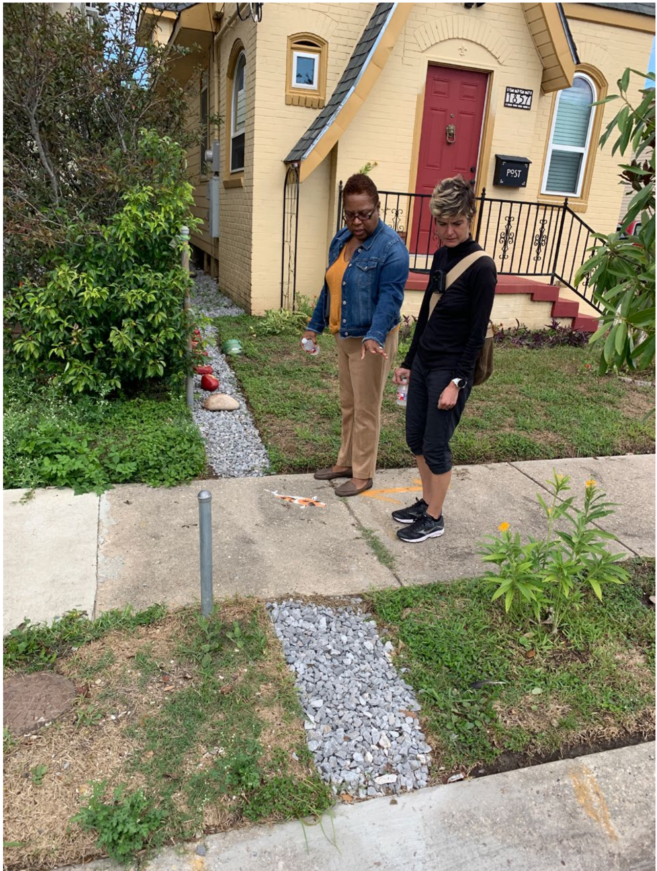
Angela shows me drainage solutions installed on her block. Image courtesy of A House Unbuilt.
